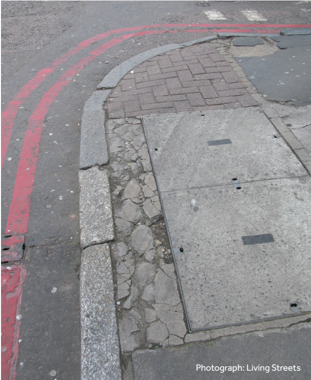
Poor quality pavement
