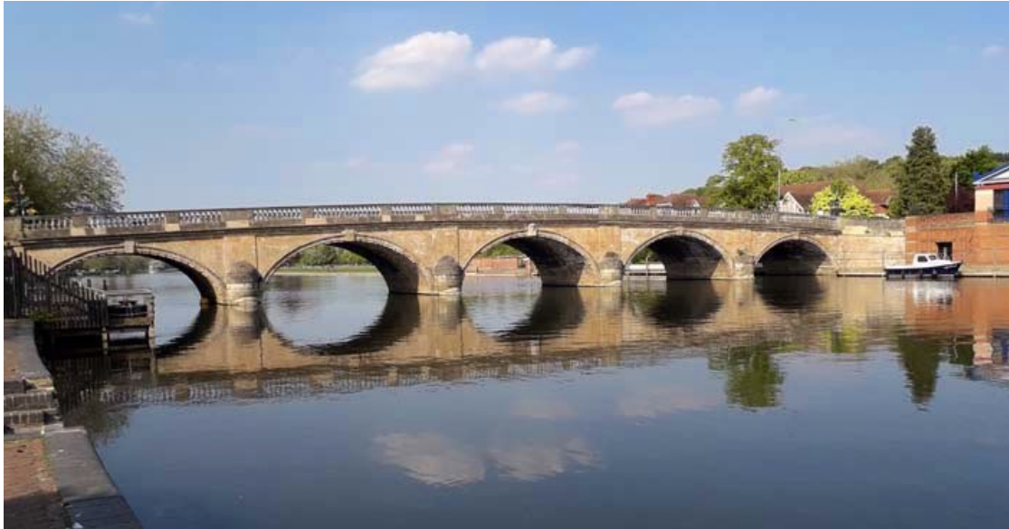
Henley Bridge, south side
