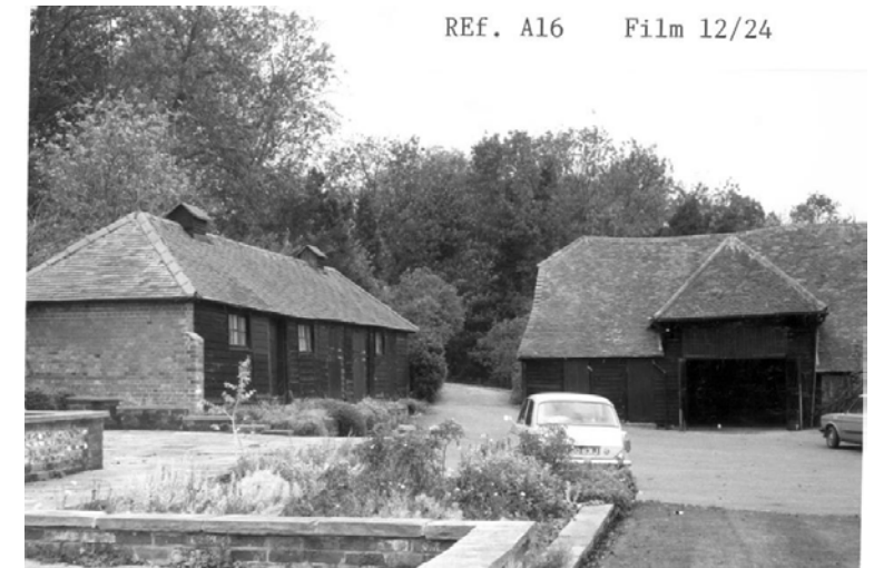
Archive image from 1980 showing the outbuilding having been demolished. Copyright NT.
