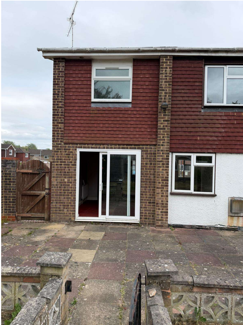
View of the existing rear elevation and garden area demonstrating the predominantly hard surfaced nature of the development footprint.
