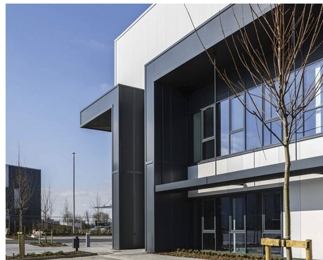
Dual aspect office fronting two elevations with fully glazed corner entrance & metal or timber bris soleil to south/west facing elevations
