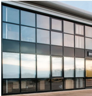
03 Full height curtain wall glazing with lookalike panels to floor zones
