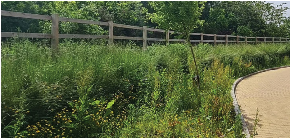
Vegetated Rootloak retaining wall cladding
