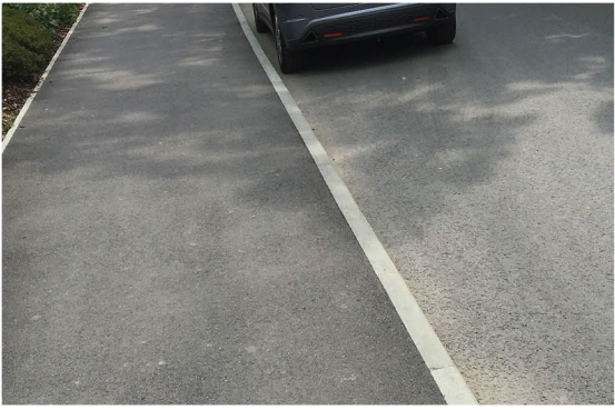
Tarmac footpath and access road
