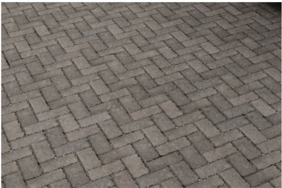
Permeable Block paving to parking bays
