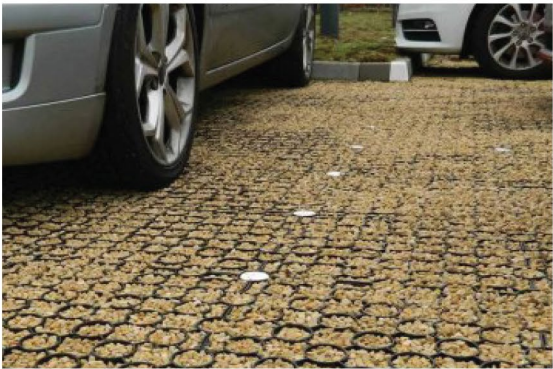
SuDpave 40 Permeable Pavers to Northern Car Park with Gravel Infill
