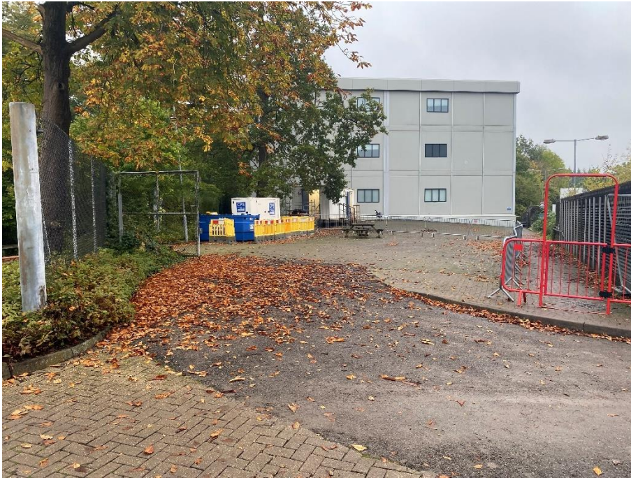
Photograph 19. Former office block
