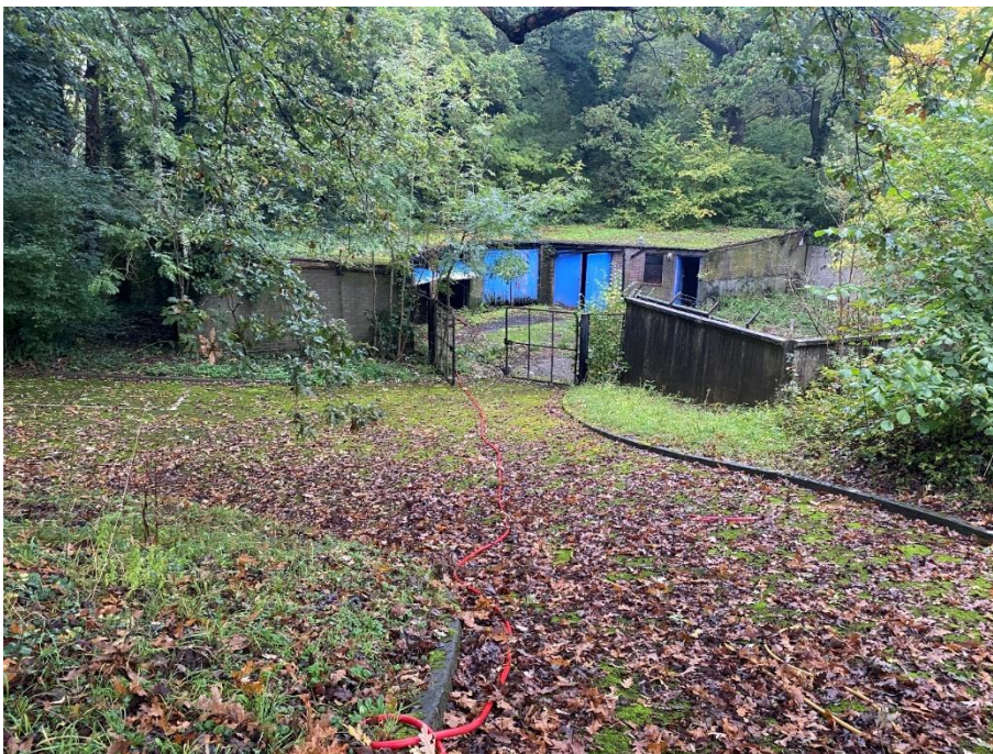
Photograph 22. Outbuildings in the northeastern extent of the Site
