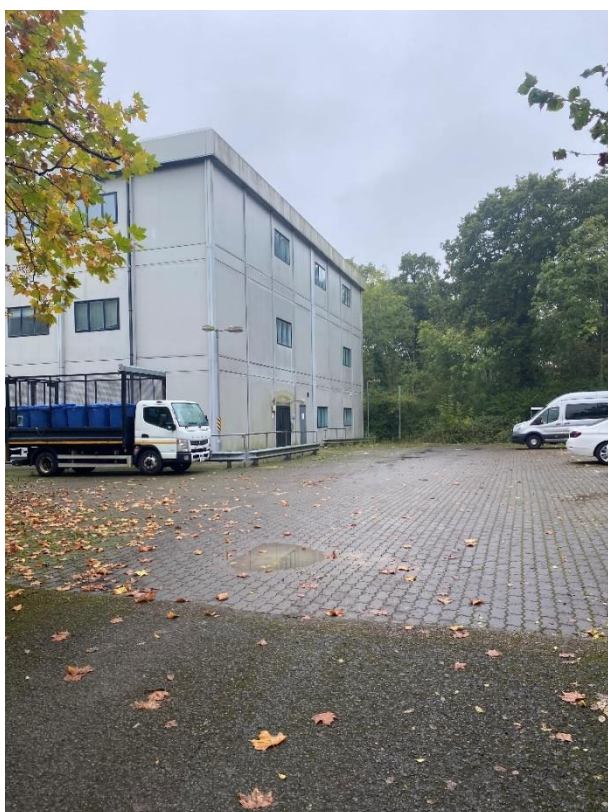
Photograph 18. Former office block
