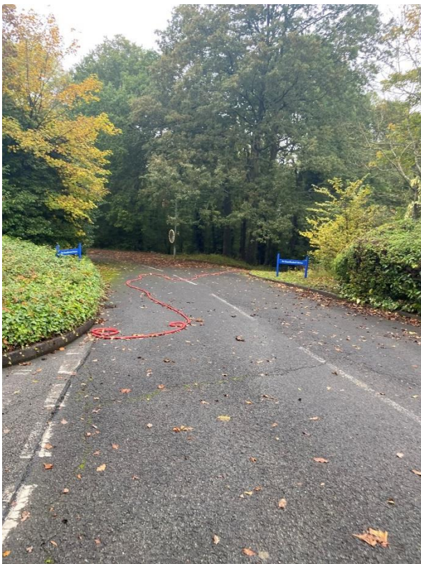
Photograph 20. Sample photograph of existing access roads
