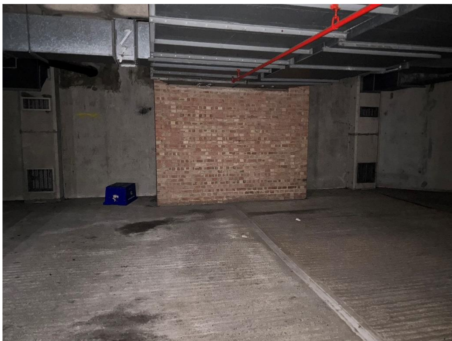
Photograph 34. Illustrative view of the basement with former openings closed
