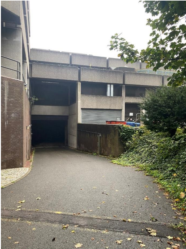
Photograph 31. Shire Hall and levelling
