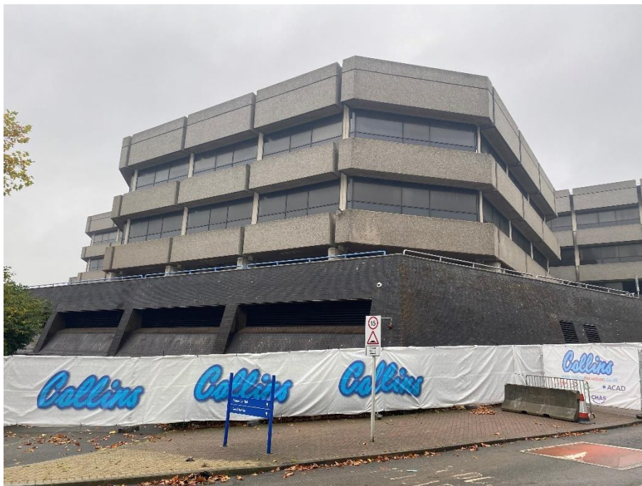
Photograph 33. Shire Hall and levelling
