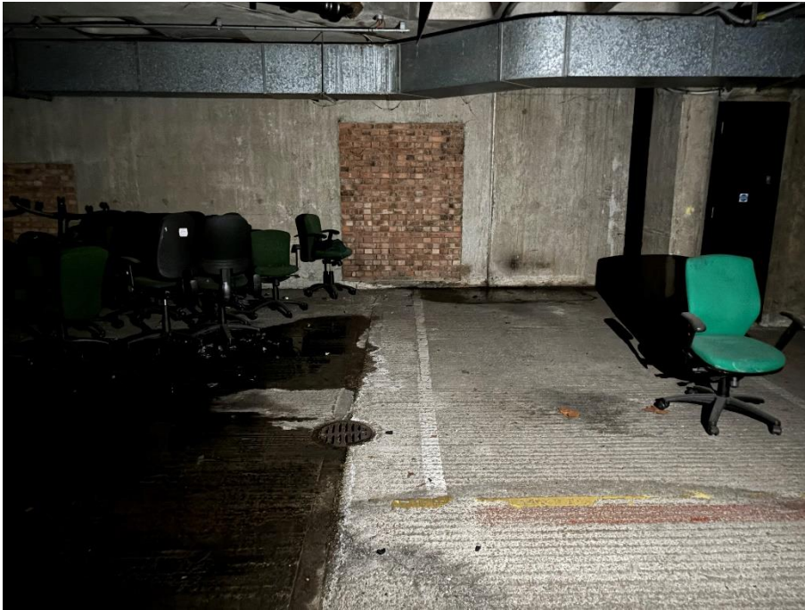
Photograph 35. Illustrative view of the basement with former openings closed
