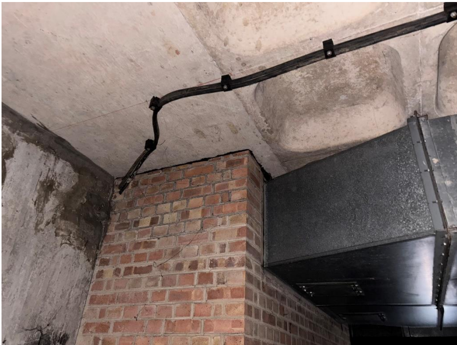
Photograph 36. Illustrative view of the basement with former openings closed
