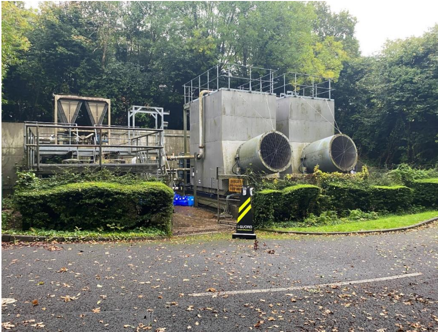
Photograph 23. Former tank infrastructure
