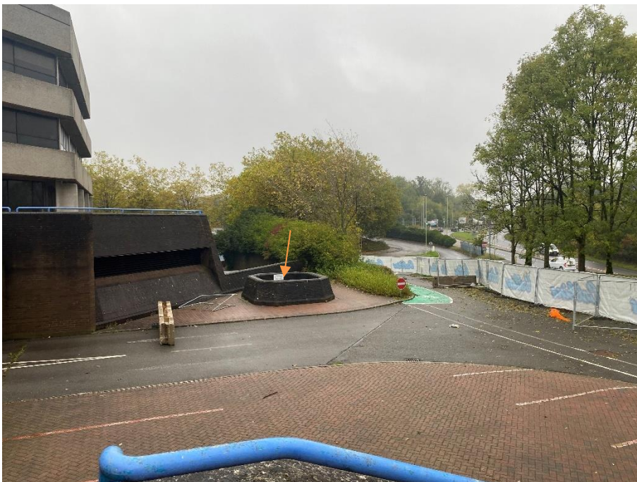
Photograph 32. Shire Hall, levelling and below ground features (demarcated by the arrow)
