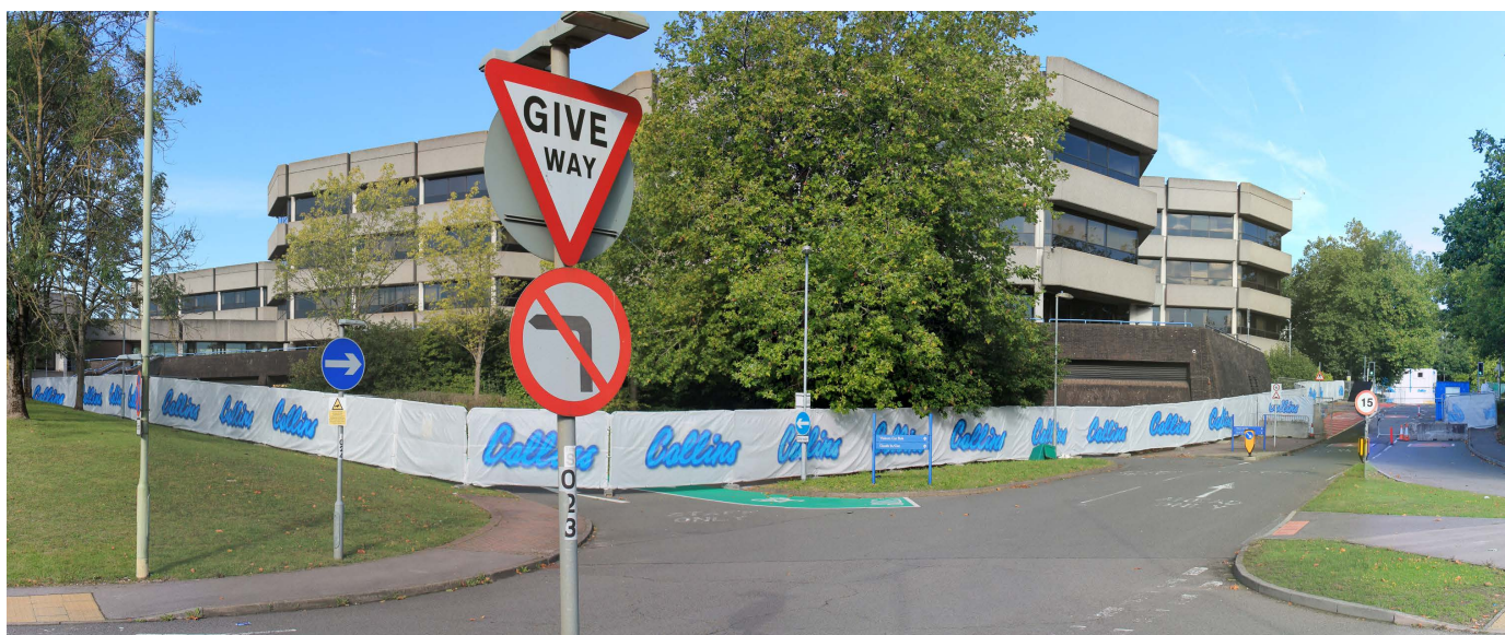
Existing site image showing office building from site entrance.
