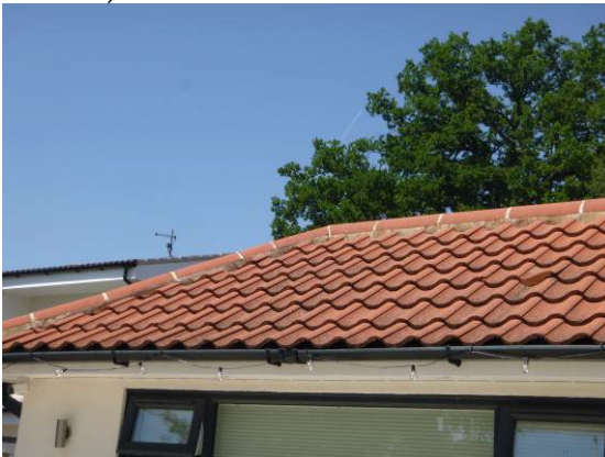
Photograph 5. Intact ridge tiles and ridge mortar (rear elevation).
