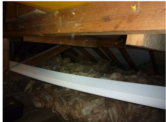
Photograph 12. Eaves filled with fibreglass.
