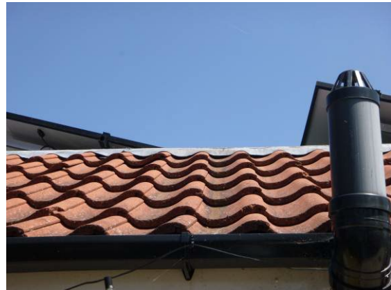
Photograph 7. Lead flashing tight to clay pantiles (western elevation).
