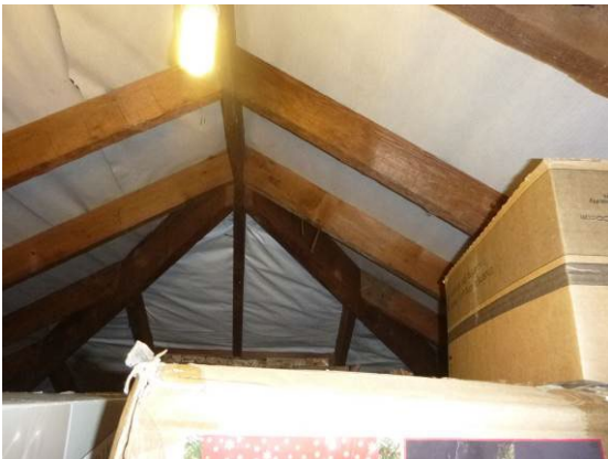
Photograph 11. Timber 'cut and pitch' construction with lightly cobwebbed ridge.
