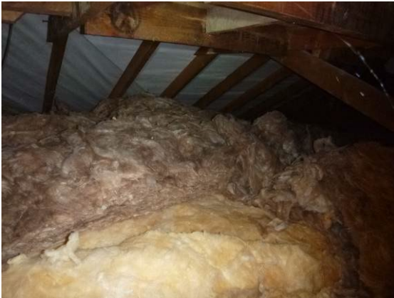
Photograph 15. Thick fibreglass insulation between joists.
