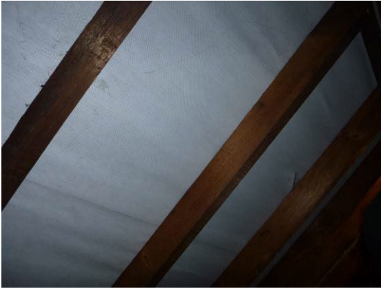
Photograph 13. Intact breathable membrane across the roof.
