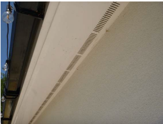
Photograph 8. uPVC soffits tight to rendered brick of the bungalow (western elevation).
