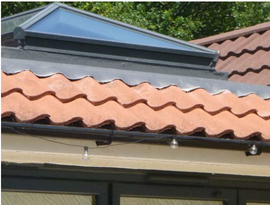
Photograph 6. Lead flashing tight to clay pantiles (rear elevation).
