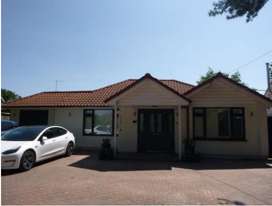
Photograph 1. Front of property viewed from north.
