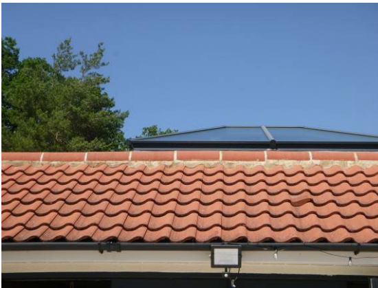
Photograph 3. Overlapping clay pantiles (rear elevation).
