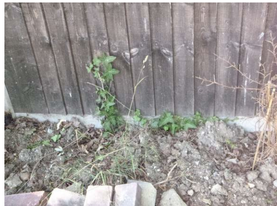
Photograph 20. Concrete gravel boards at base of garden fences.
