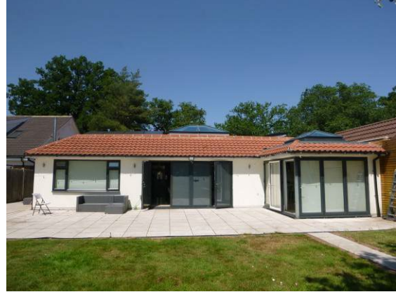
Photograph 2. Rear of property viewed from south.
