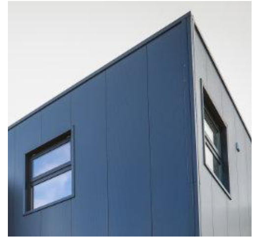
04_Togher Modular Primary School, Meitheal Architects, Ireland
