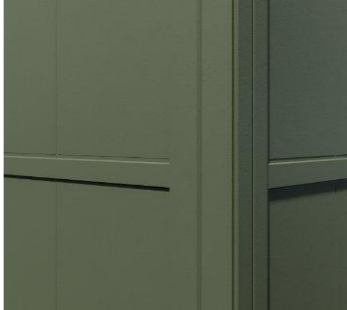
02_Corner flashing
