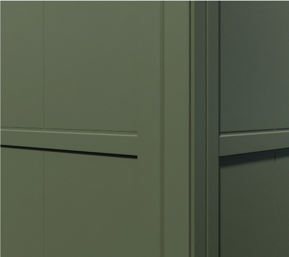
02_Corner flashing
