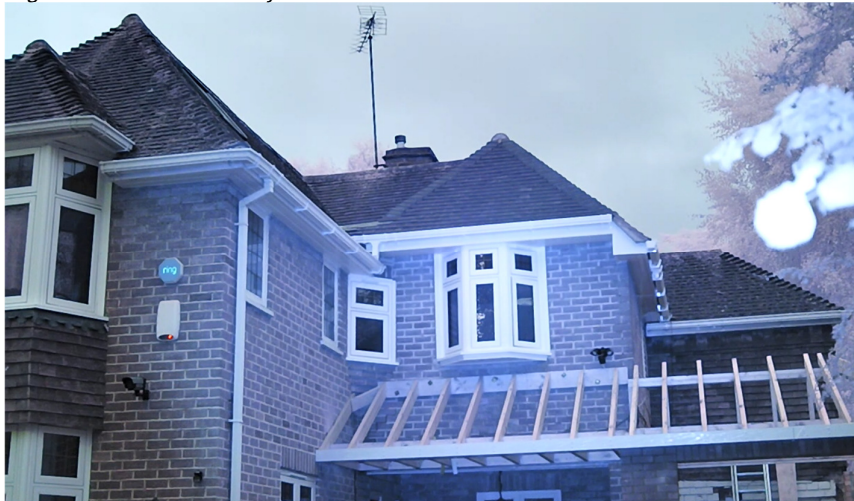
Sionyx Aurora Pro at Survey Location 1 on 9 th July 2024
