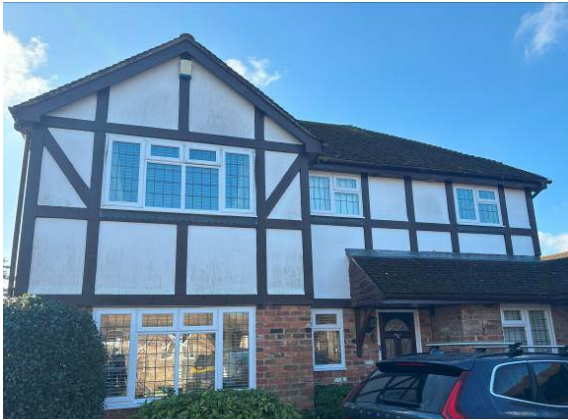
Photograph 1. Front of the house viewed from the north.
