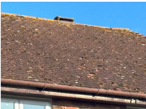
Photograph 4. Roof tiles all in place, flat and tightly fitted on the main roof.
