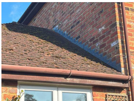
Photograph 8. Lead flashing tight at the junction of the single storey extension with the main house.
