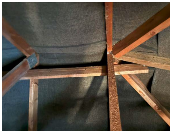
Photograph 16. Bitumen felt intact throughout the void and the ridge was lightly cobwebbed.
