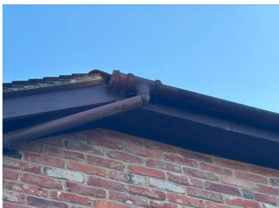
Photograph 7. Soffits tight along the eaves at the western side of the house.
