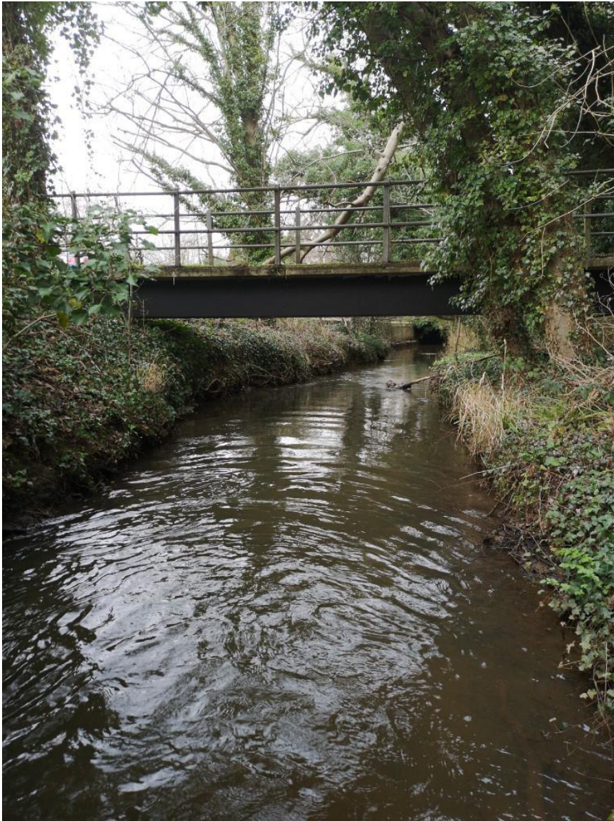
Figure 2-7 Bridge upstream of weir pool at downstream end of site
