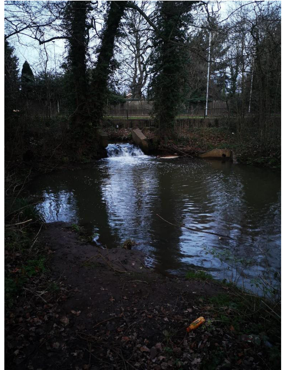
Figure 2-8 Weir, weir pool and small culvert outflow (view upstream)
