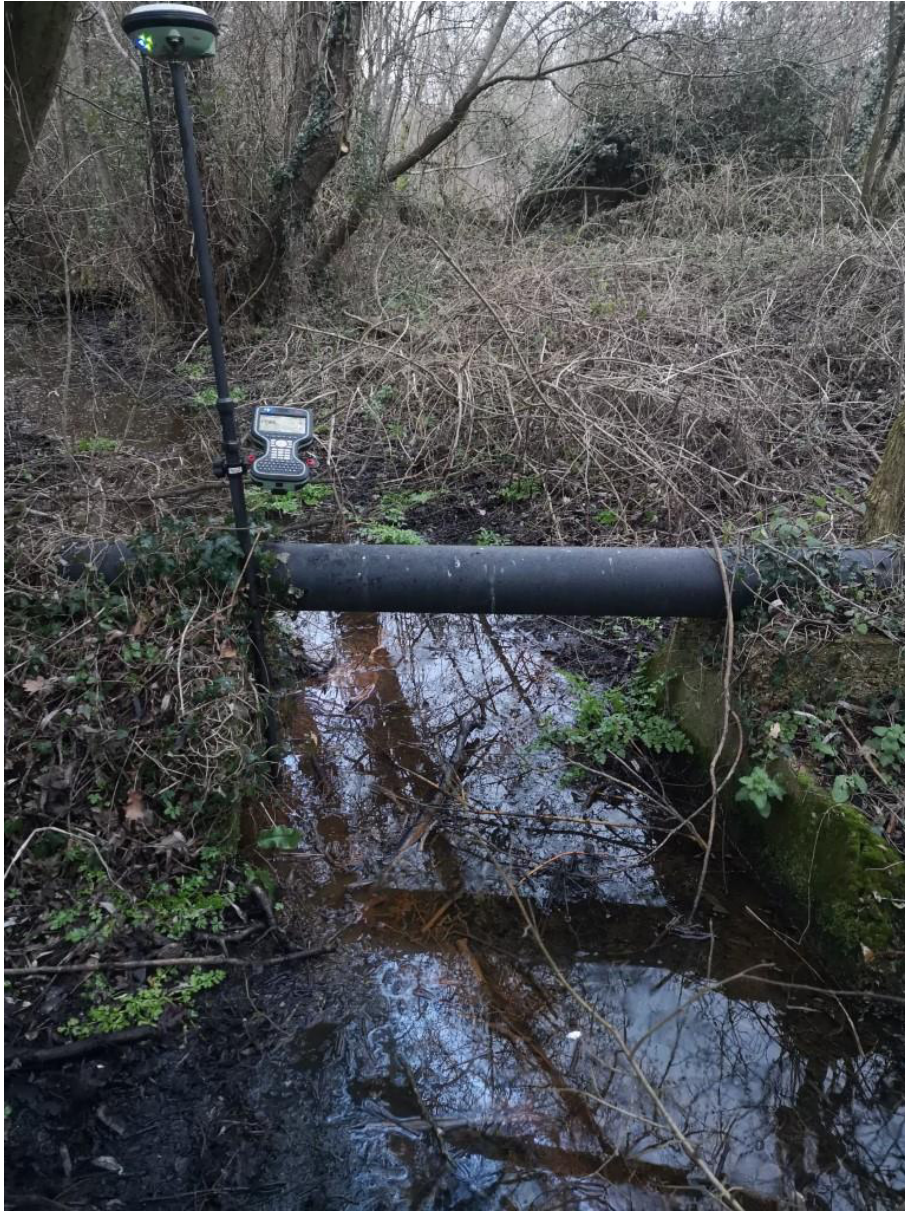
Figure 2-5 Second foul sewer pipe and abutments, in historic channel
