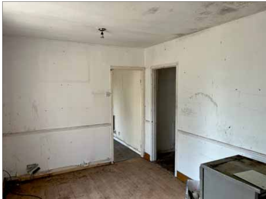
Photograph 3: Showing the internal structure of one of the buildings.
