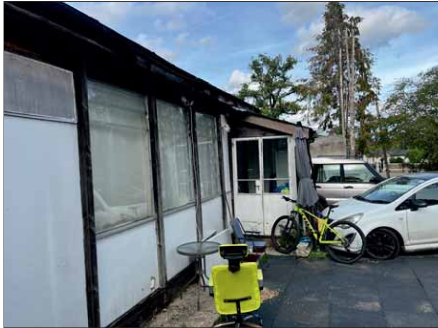
Photograph 2: Showing the front of the existing buildings.
