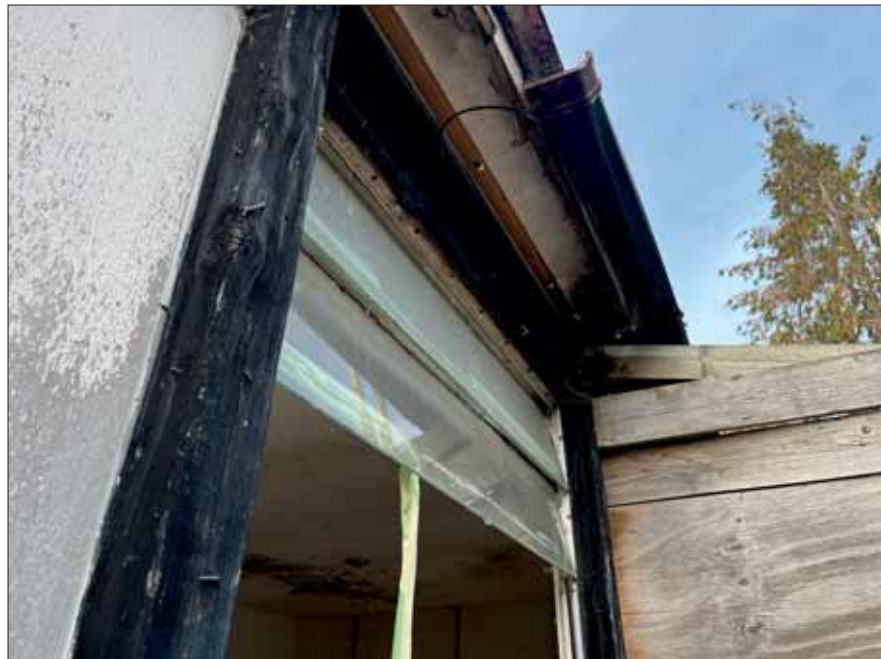
Photograph 4: Showing a close-up inspection of the front exterior on one of the buildings.
