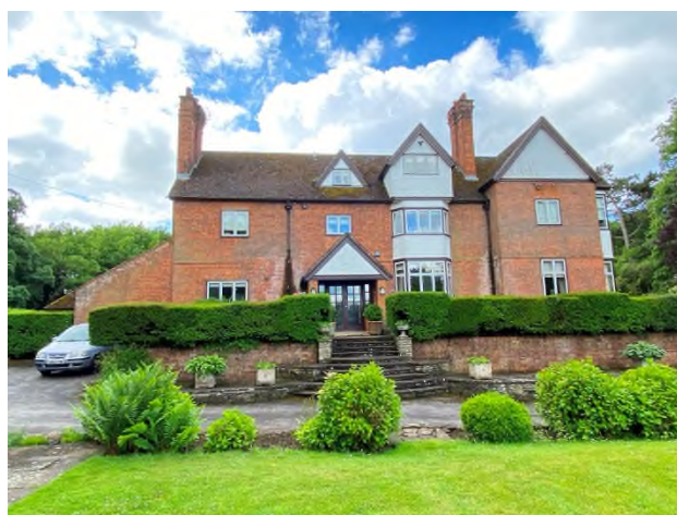
Figure 1: North elevation of Aston Rise
