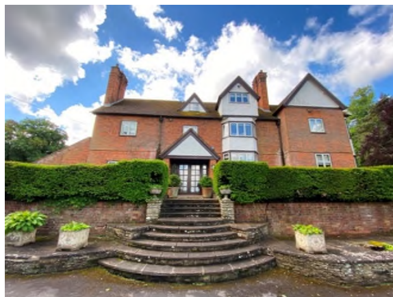
Figure 13: North elevation of Aston Rise
