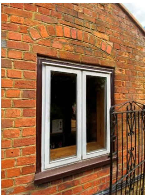
Figure 24: Original window opening on the south elevation of the lean-to
