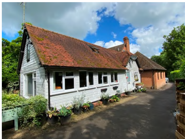
Figure 17: Oblique view of 'the cottage' looking north-west
