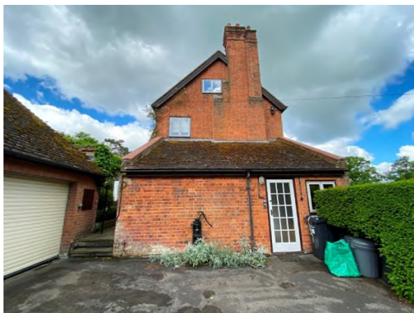
Figure 16: East elevation of Aston Rise
