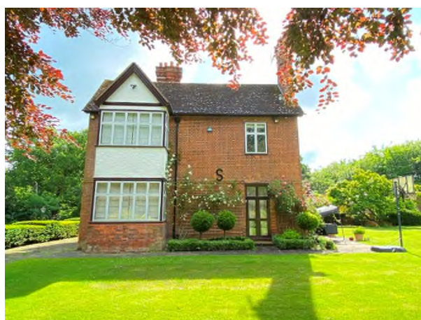
Figure 15: West elevation of Aston Rise
