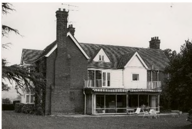
Figure 11: South elevation of Aston Rise in 1980
