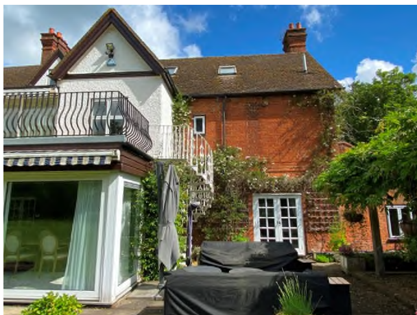
Figure 26: Right hand side of the south elevation
