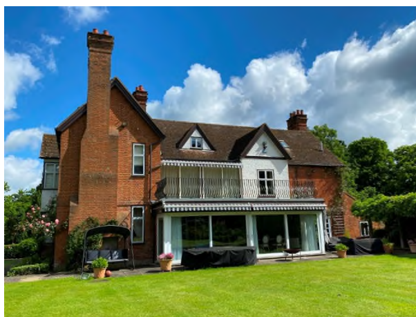
Figure 14: South elevation of Aston Rise
