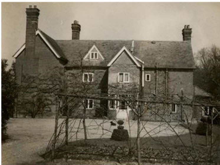
Figure 6: South elevation of Aton Rise in 1948
