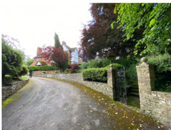
Figure 12: Oblique view of the north and west elevations of Aston Rise on the approach to the house along the drive
