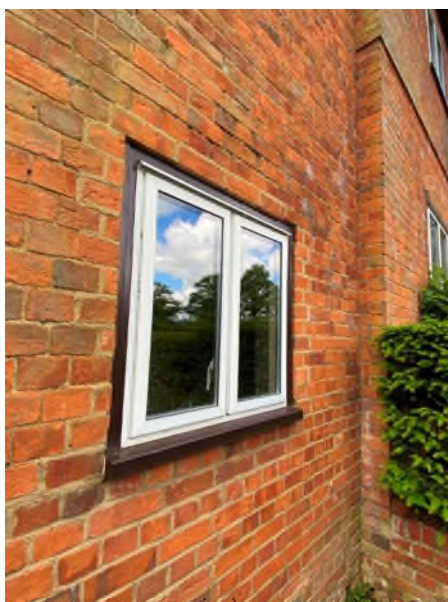
Figure 22: Later or modified window opening on the north elevation of the lean-to
