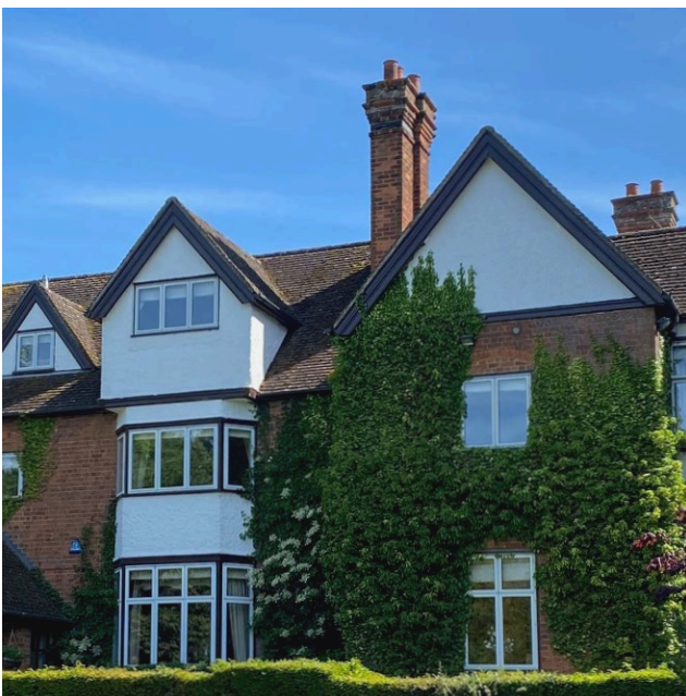
Figure 19. Existing Bay Window & Rendered Gable to Front
