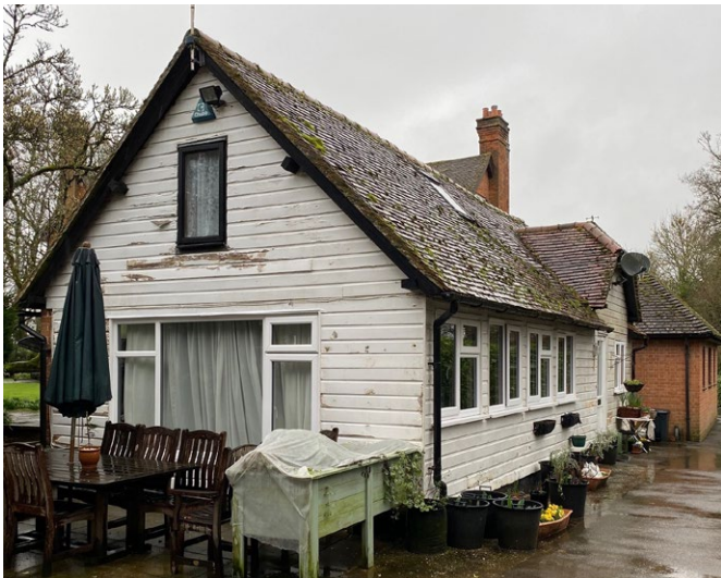
Figure 22. Existing side view of cottage towards workshop
