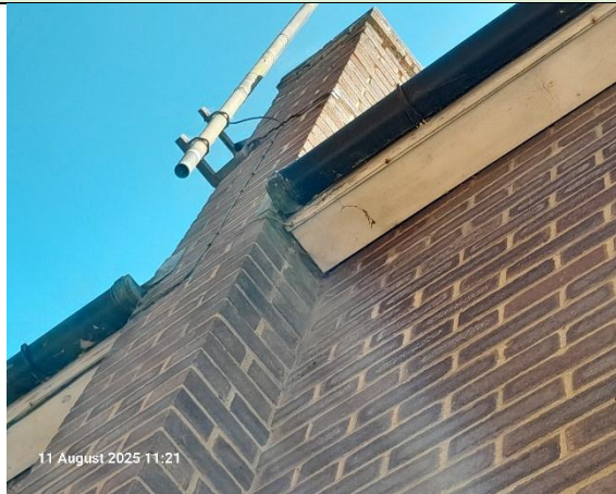
Figure 3: Well sealed soffit boxes
