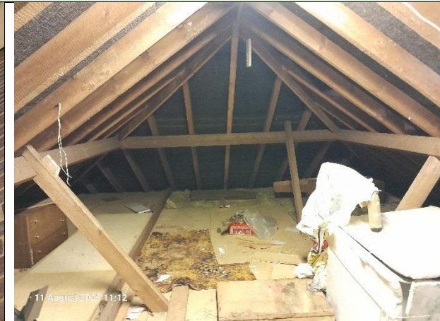
Figure 4: Loft void within B1.
