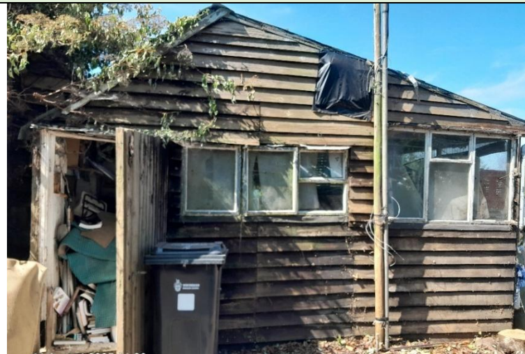
Figure 9: The front of B2b
