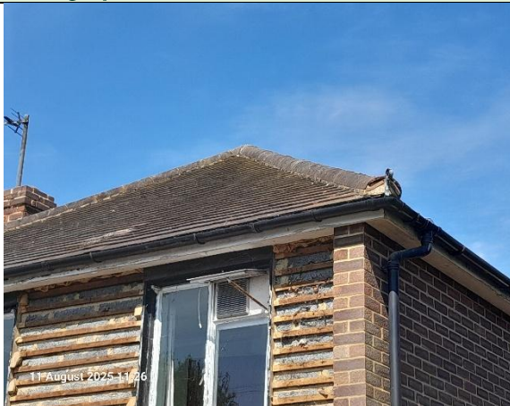
Figure 2: Roof tiles and removed hanging tiles.
