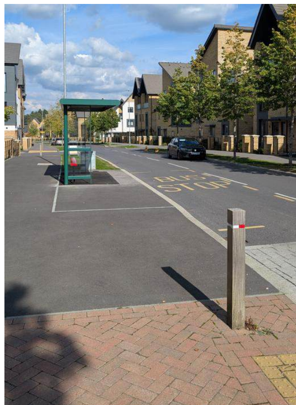
Photograph 12: Buckler's Ride Bus Stop
