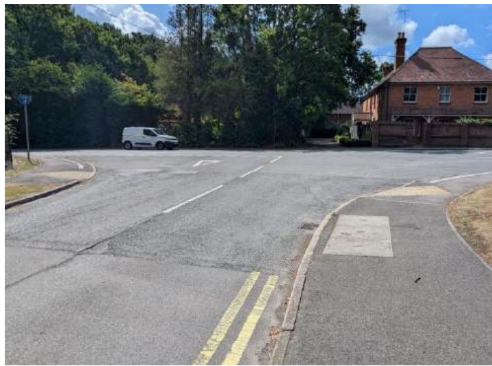
Photograph 1: Existing Site Access
