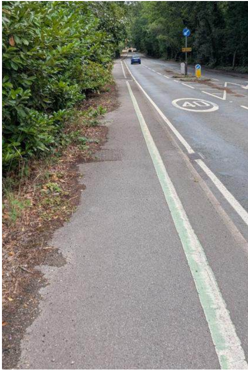
Photograph 6: Nine Mile Ride Shared Footway/Cycleway (facing east)
