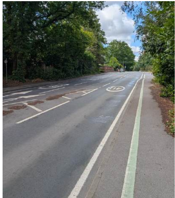
Photograph 5: Nine Mile Ride (facing west)
