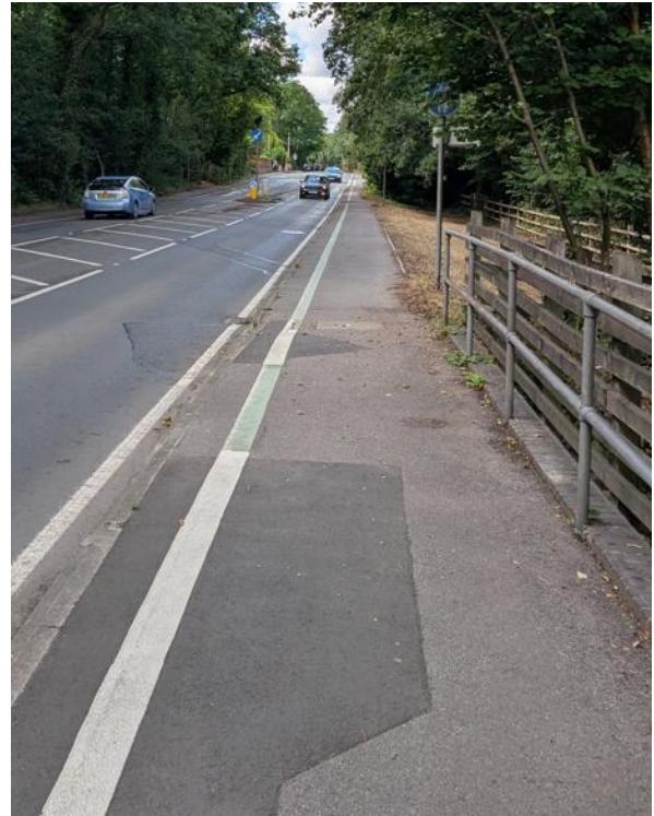
Photograph 7: Nine Mile Ride Shared Footway/Cycleway (facing west)
