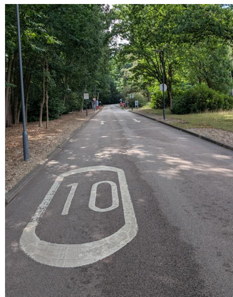
Photograph 3: Site Access Road (facing south)
