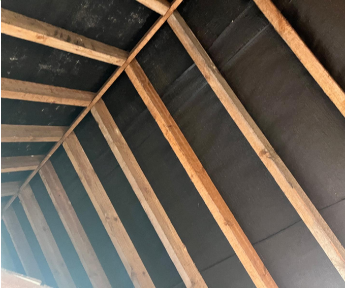
Inside the loft
