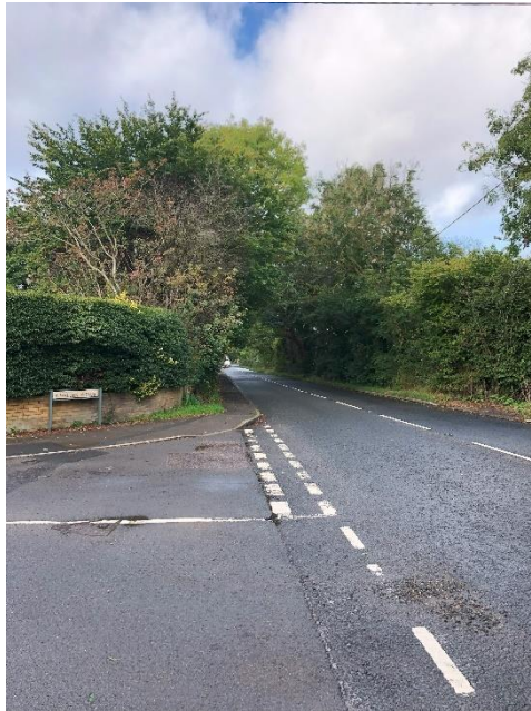
Photograph 3: Reading Road Footway Facing west
