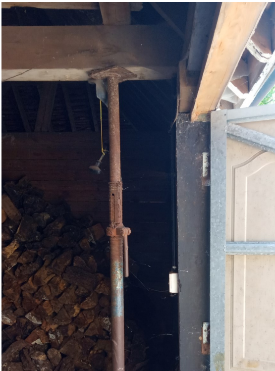
F) Acro prop to support existing lateral beam
