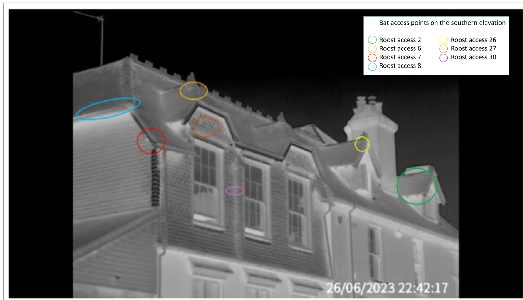
Figure 6: Annotated photographs of roost access locations for three elevations
