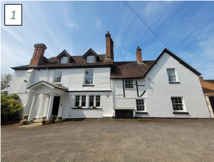
Figure 7: Photos of the site
