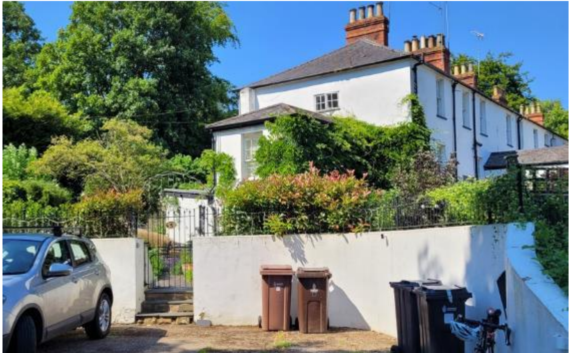
Property as viewed from Aston Lane
