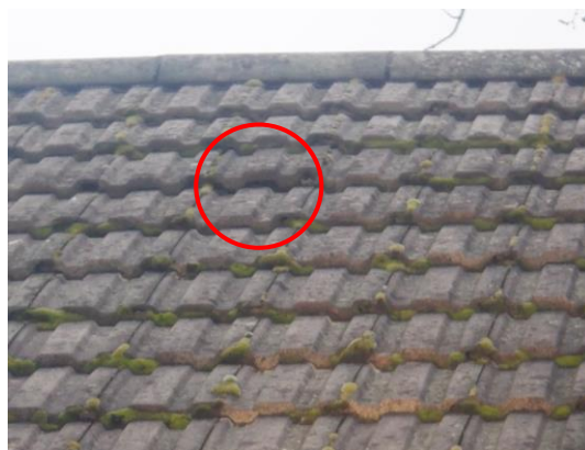
Photograph 4. Lifted interlocking tile; intact dry-fixed ridge tiles (southern elevation).
