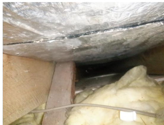
Photograph 12. Open eaves (roof void).
