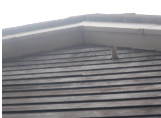
Photograph 9. Tight timber cladding and intact sealant along soffit (eastern elevation).
