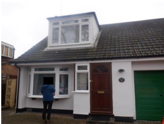
Photograph 1. Front of house viewed from south.
