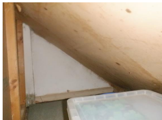
Photograph 16. Intact plasterboard on ceiling and boarding with carpet on floor (eaves space).
