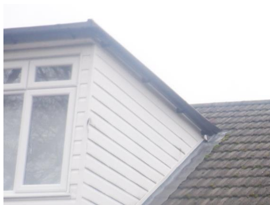
Photograph 6. Tight cladding on dormer (southern elevation).
