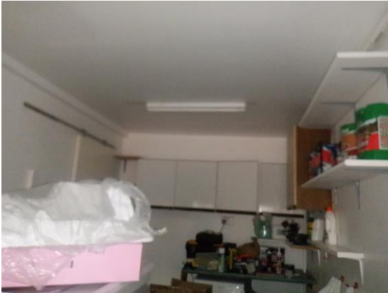
Photograph 17. Painted plasterboard internally (garage).
