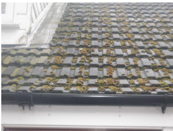
Photograph 3. Tight interlocking roof tiles (northern elevation).
