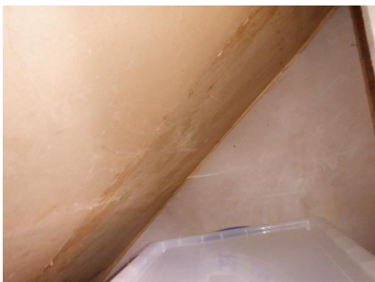
Photograph 15. Intact plasterboard on ceiling and side (eaves space).
