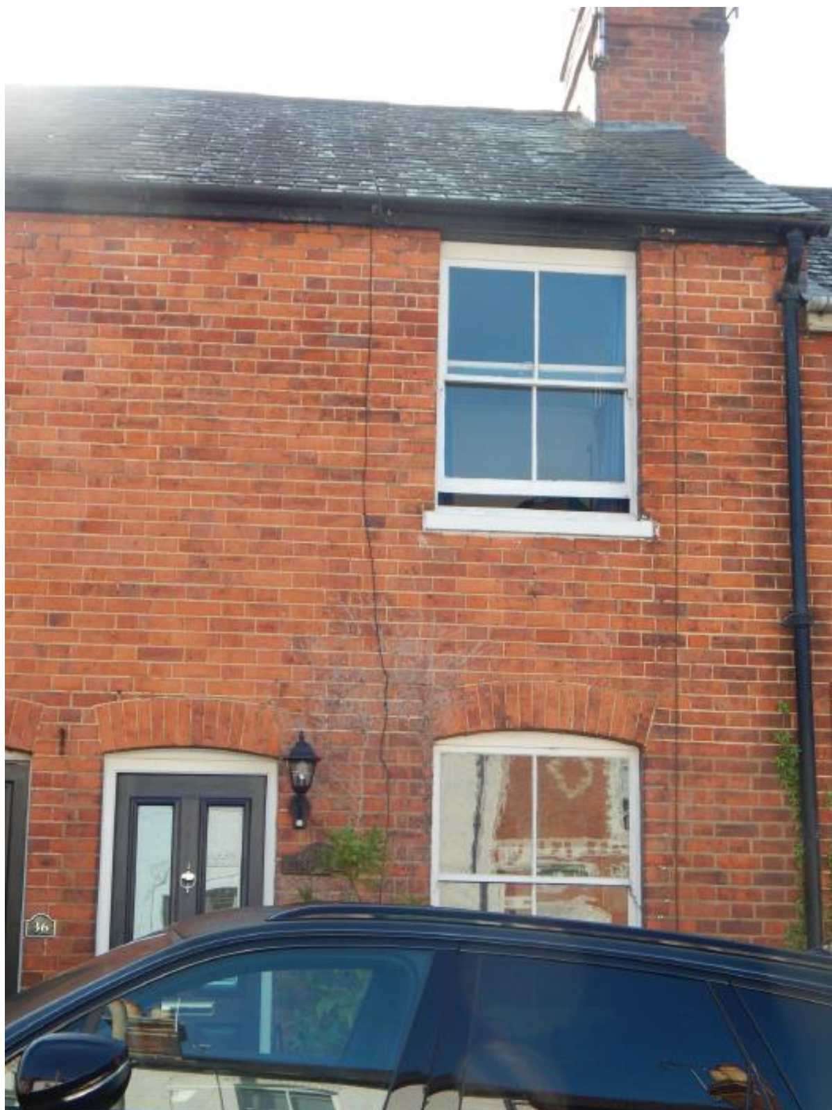
Image 1 – Front North/West facing elevation of the property
