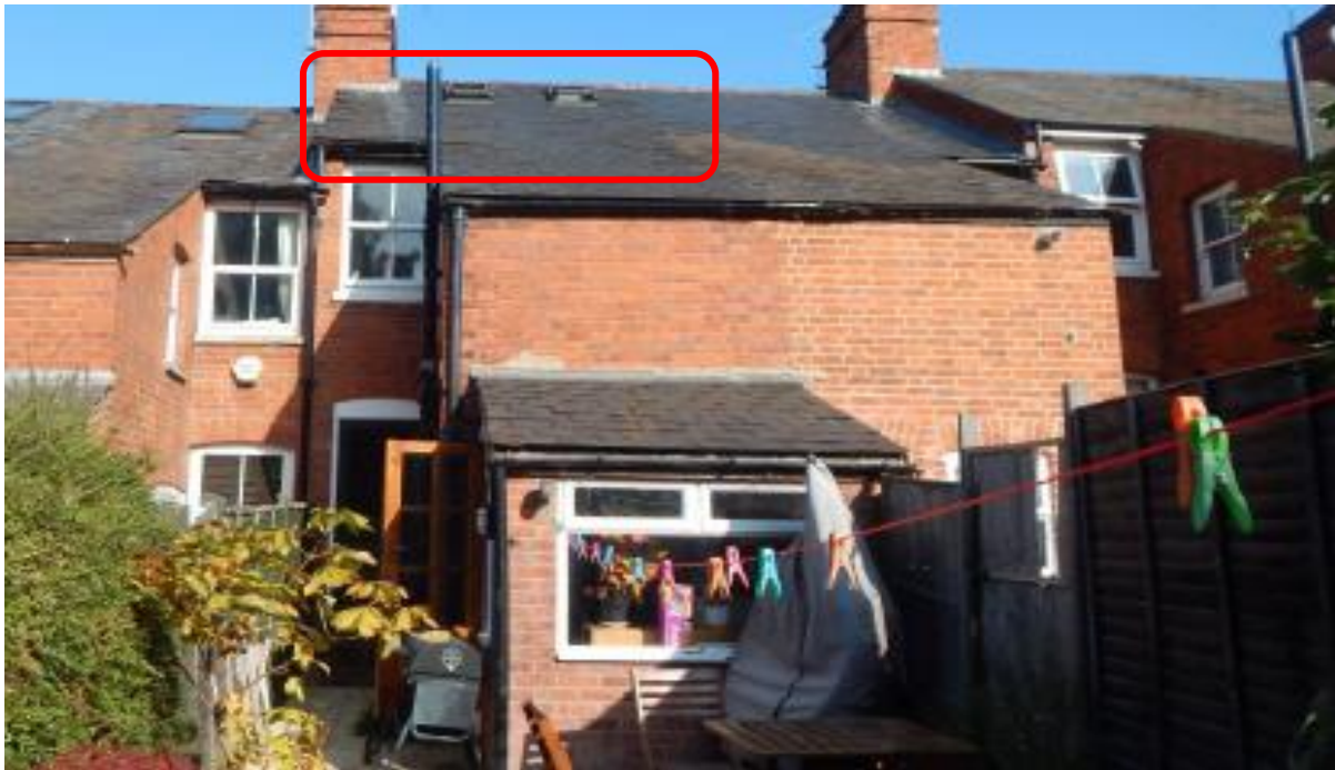
Image 2 – Rear elevation of the property where a number of gaps of adequate proportions to offer shelter opportunities for bats were observed
