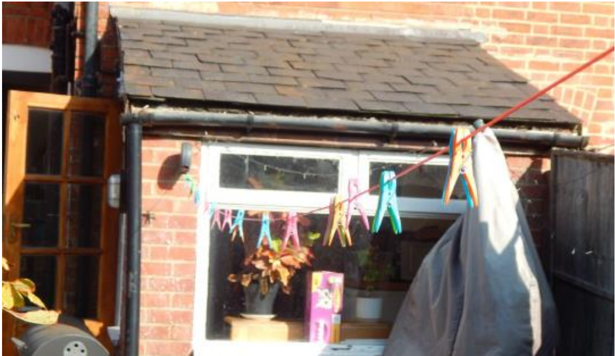
Image 4 – Lower rear section of the property
