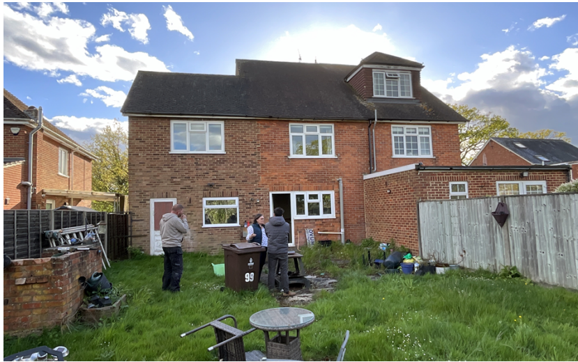
Image 1 – Rear elevation of property with neighbouring property in view.
