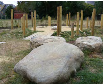
PLAY BOULDERS Proposed play boulders to be naturally smooth or have a slightly rough surface with no sharp edges. Stone must not be slippery when wet. To be sustainable sourced – locally where possible. To be set 1/3 into the ground.
