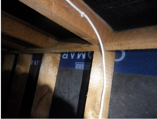
Photograph 9. Breathable roofing membrane and bitumen felt
