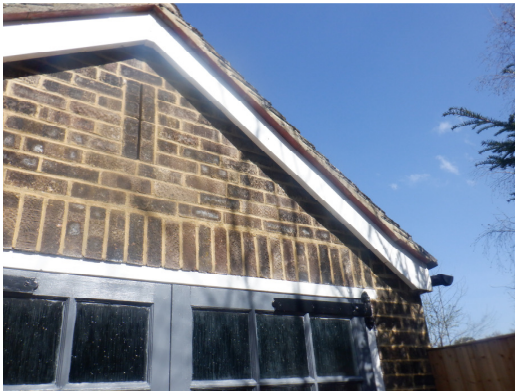
Photograph 8. Garage with tight barge boards.
