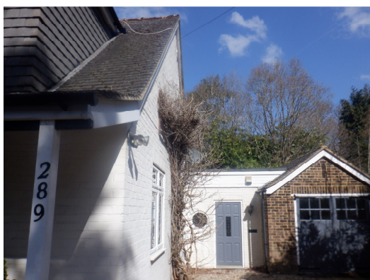
Photograph 3. Garage attached to the eastern side of the house.
