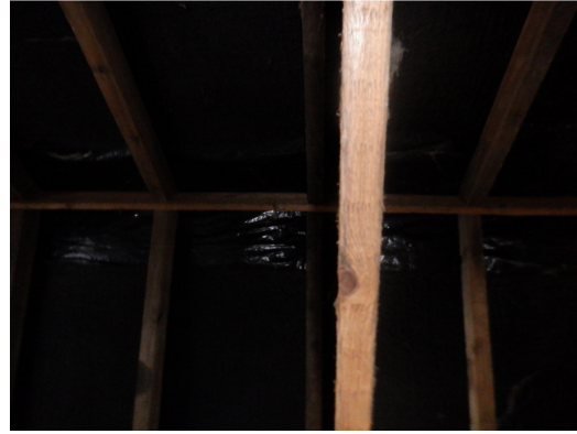
Photograph 13. Plastic roof sheeting
