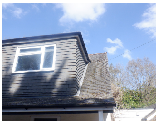
Photograph 4. Tight/flat plain roof tiles and hanging tiles on dormers
