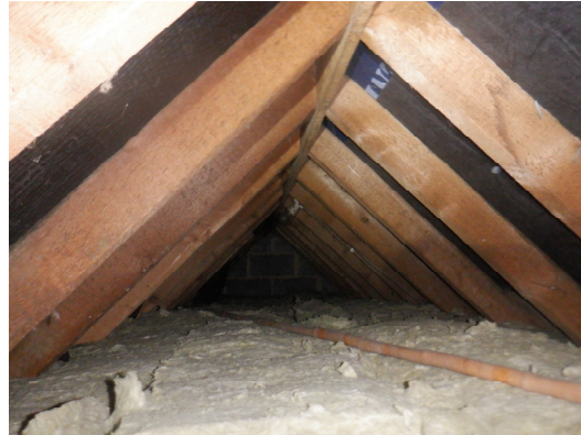
Photograph 10. Thick fiberglass insulation and no tears in roof lining or gaps in brick work
