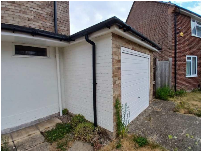
Southwestern elevation of B2.
