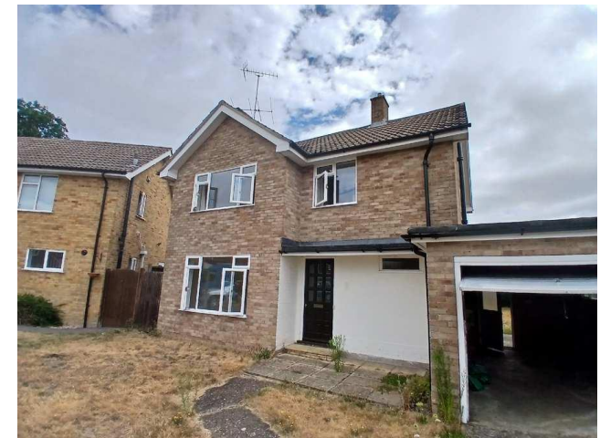
Southern elevation of B1.
