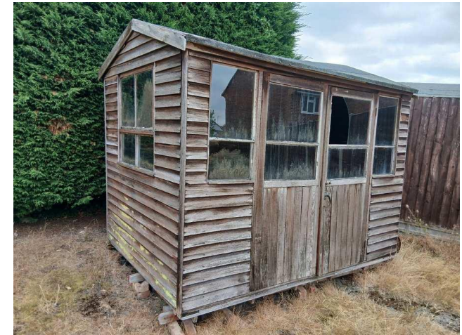
Southwestern elevation of B3.
