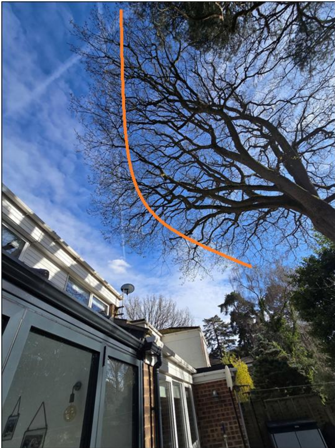
Photo 1 – T001 (Oak) – Indicative line of proposed reduction on western half of tree to create reasonable clearance to rear elevation of 15 Heathermount Drive
