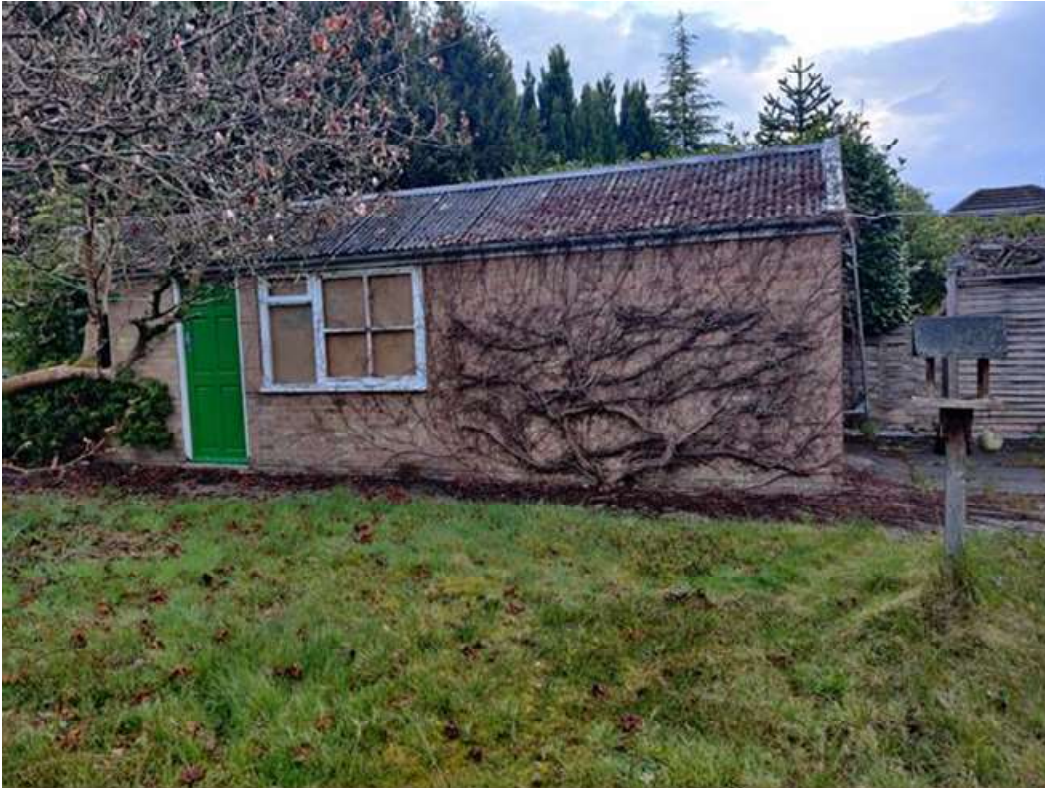
Photograph 5: Garage Building B2.
