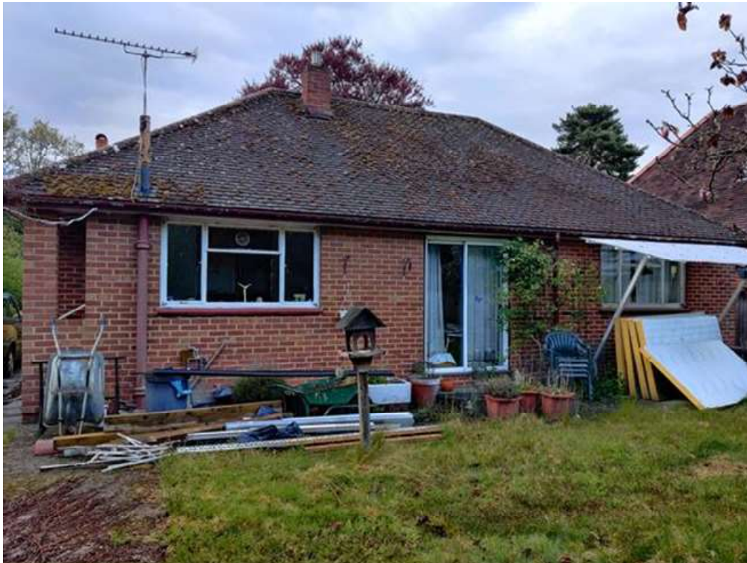
Photograph 1: View of B1 from the south.
