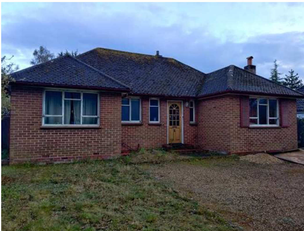
Photograph 2: View of B2 from the north.
