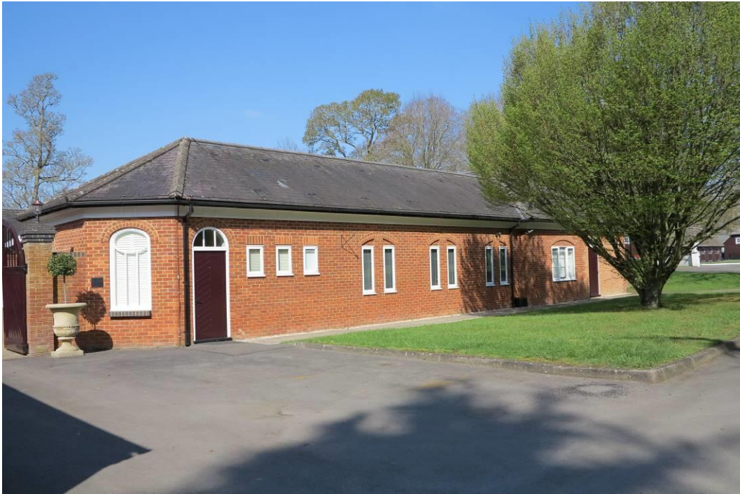
Plate 21. Extensions to the rear of the listed stable complex
