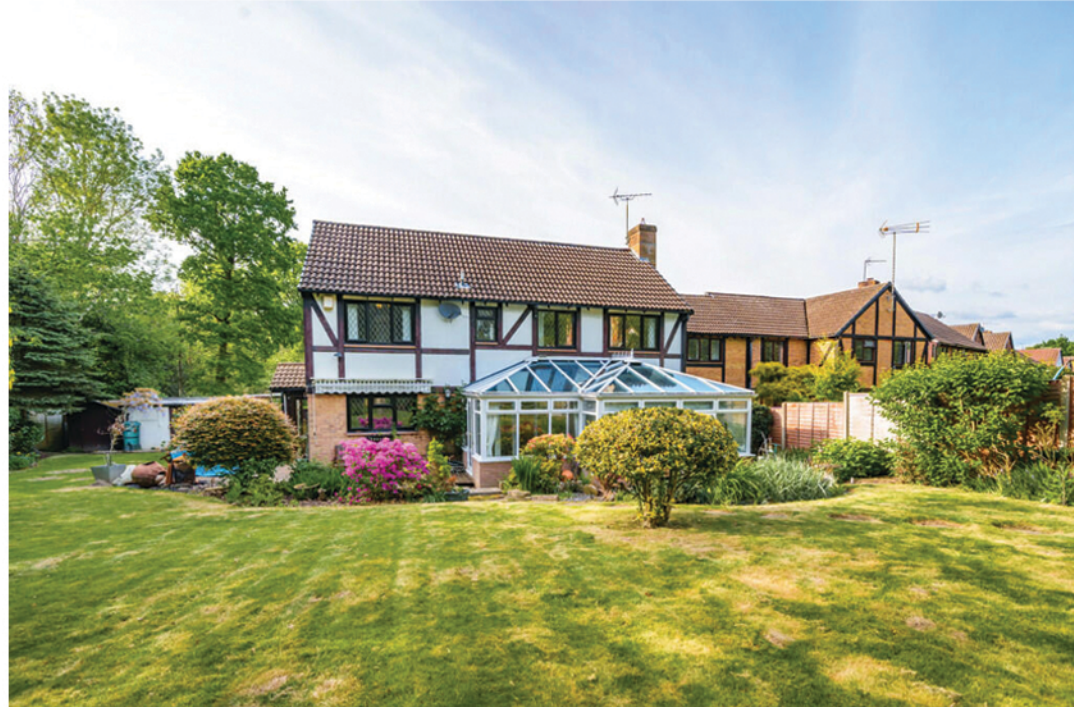
REAR ELEVATION PHOTO
