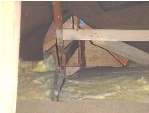
Photograph 13. Dormer timber boarded gable (roof void).
