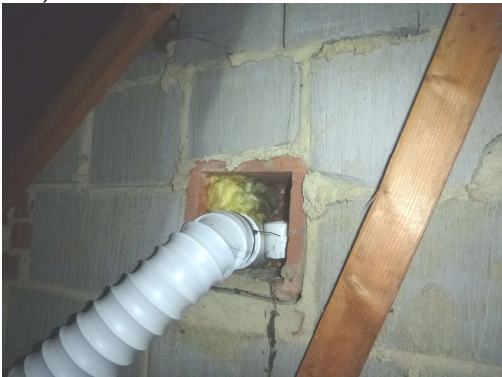
Photograph 15. Extraction tube secured to vent brick with some spray foam present on the southern gable (roof void).
