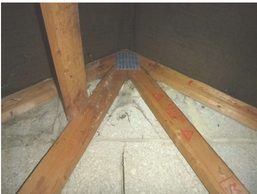
Photograph 20. Cobwebbed blockwork northern gable (roof void).
