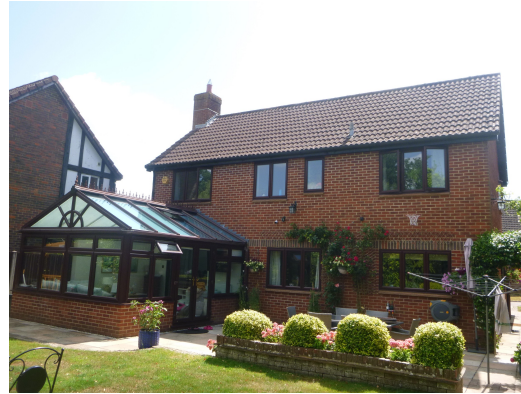
Photograph 2. Rear of property viewed from south.
