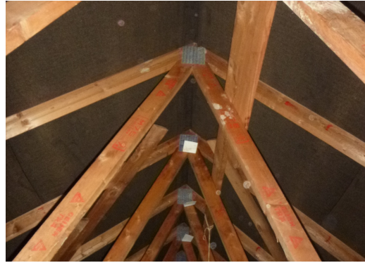
Photograph 12. Intact bitumen roofing felt (roof void).
