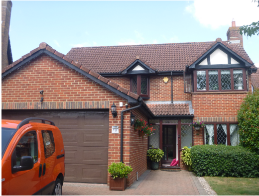
Photograph 1. Front of property viewed from north.
