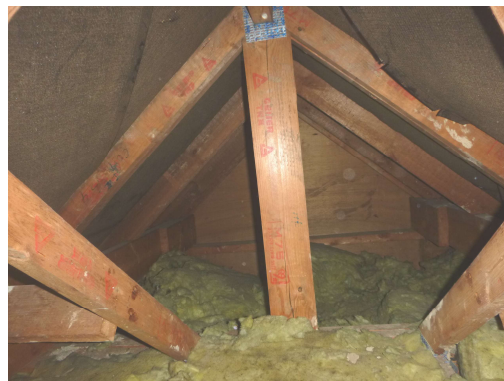
Photograph 10. Front gable extension (roof void).
