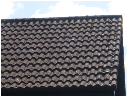
Photograph 3. Tight interlocking roof tiles (rear elevation).
