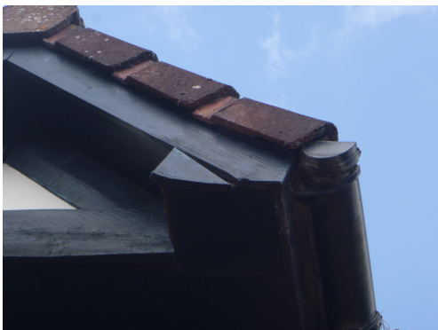
Photograph 5. Verge cap tiles tight to the fascia (front elevation).
