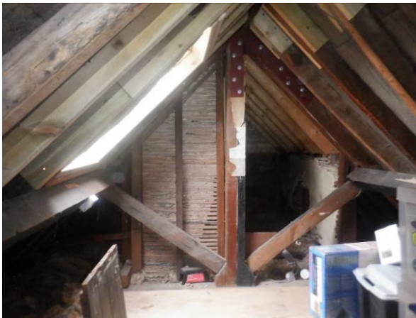
Photograph 18. Lathe, plaster and timber board cladding towards western elevation with Velux window
