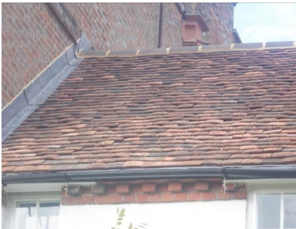
Photograph 9. Flat lead flashing (southeastern rear elevation).
