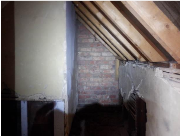
Photograph 20. Southwestern gable with brickwork, lathe and plaster.
