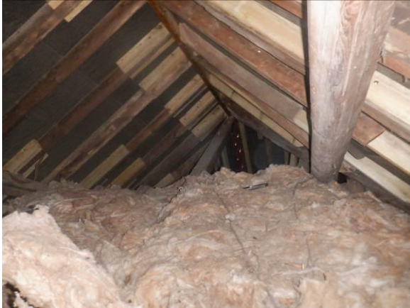
Photograph 14. 'Cut and Pitch' roof construction with supporting batons against the ridge
