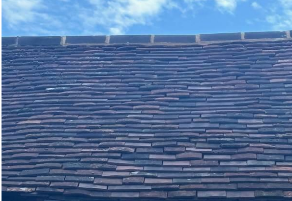
Photograph 7. Ridge mortar intact (northwest front elevation)
