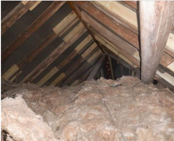
Photograph 16. Thickly packed fibreglass insulation
