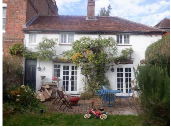
Photograph 2. Rear of property viewed from the southeast.
