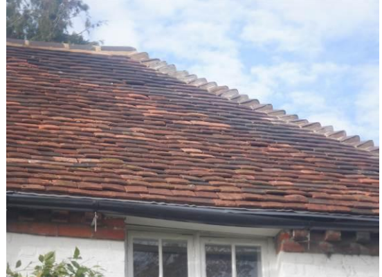
Photograph 8. Full mortared hip tiles (southeastern rear view)
