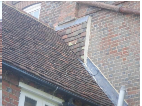
Photograph 10. Hanging tiles on adjacent property (front elevation).
