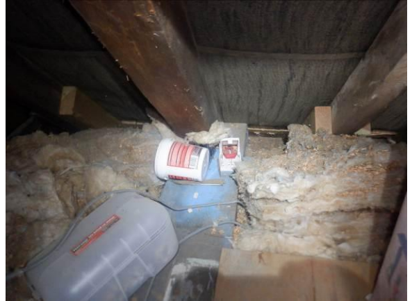
Photograph 15. Tightly fitted roofing bitumen
