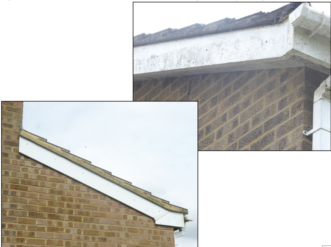
Figure 10. Example of sealed soffits/fascias. 21 Langhams Way, Wargrave. 20.08.24
