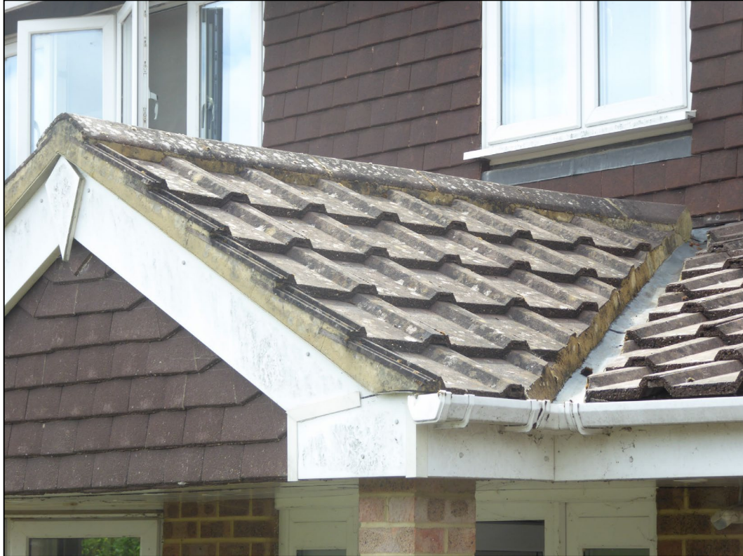
Figure 7. Example of sealed tiles/valleys/lead flashing on front porch/mono pitched roof. 21 Langhams Way, Wargrave. 20.08.24
