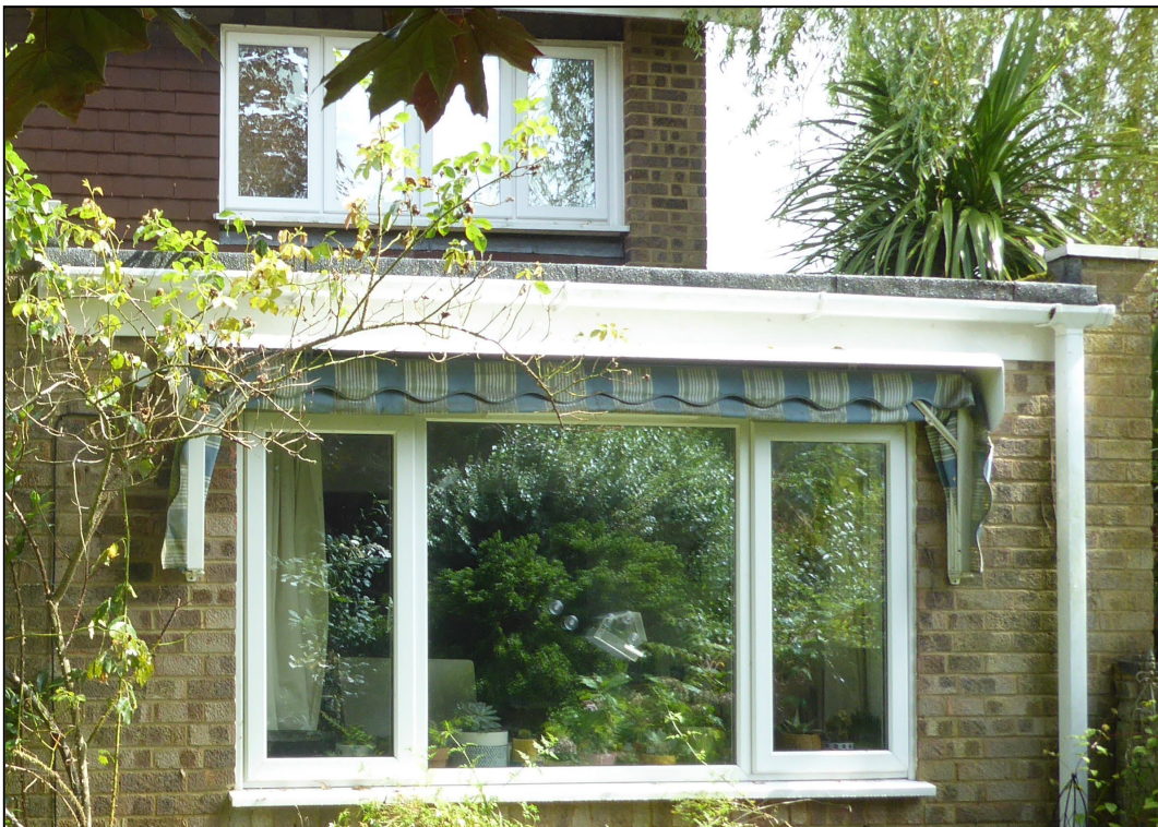
Figure 6. Single storey rear extension and bitumen covered flat roof. 21 Langhams Way, Wargrave. 20.08.24
