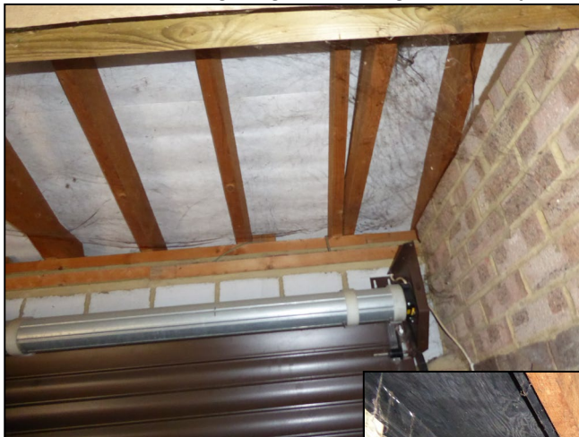
Figure 12. Example membrane on false pitched section of garage roof and example flat roof section of garage. 21 Langhams Way, Wargrave. 20.08.24
