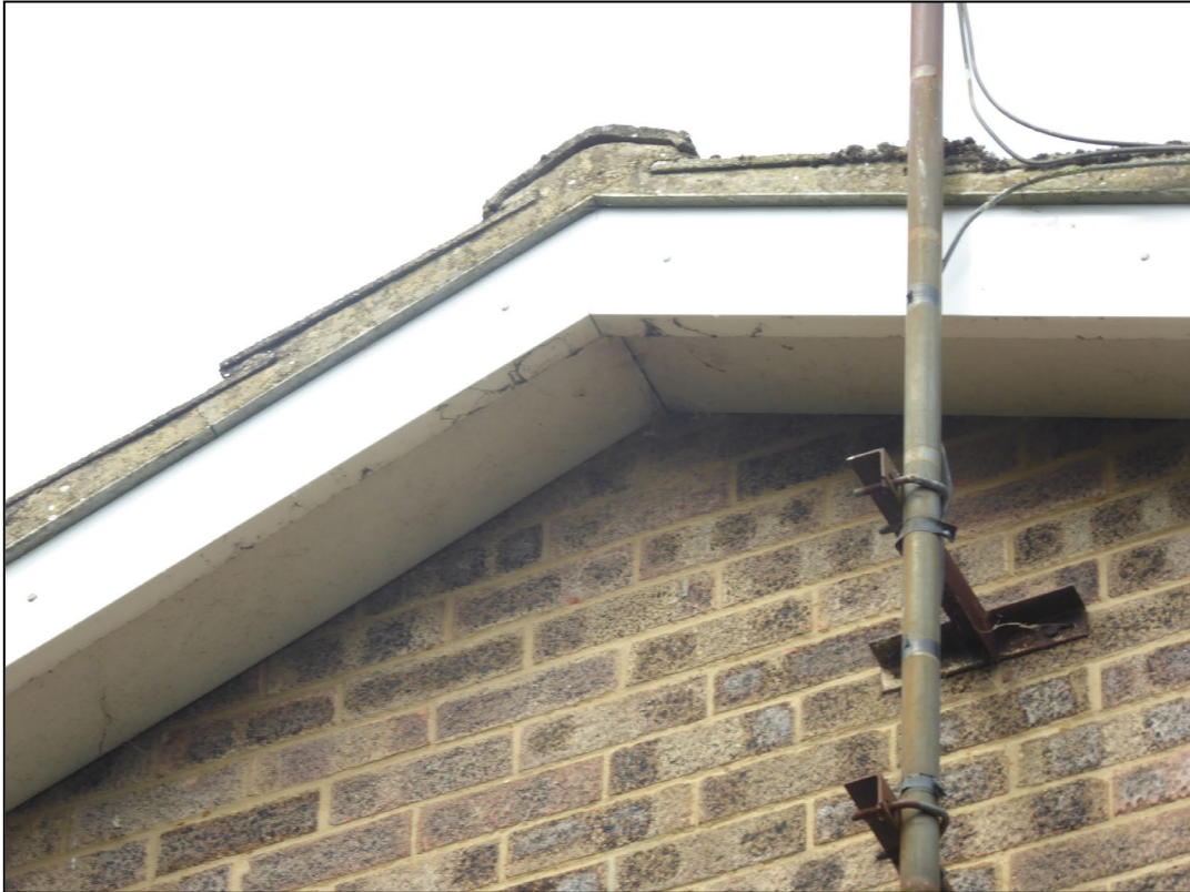
Figure 5. Example of sealed verges. 21 Langhams Way, Wargrave. 20.08.24
