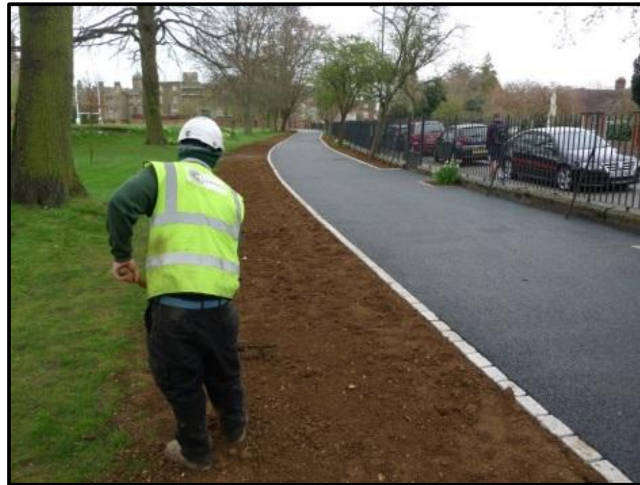
Fig 13 – In the event of 'making good' topsoil will be BS3882 compliant and raked out by hand to no greater depth than 100mm.
