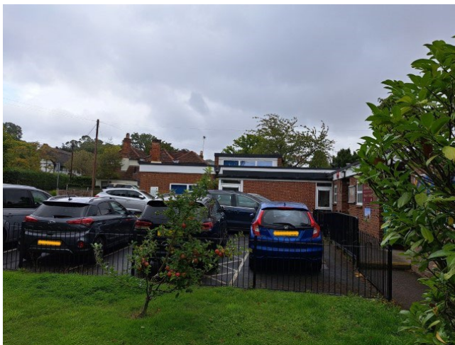
Photo 6 – View of side elevation (west)
