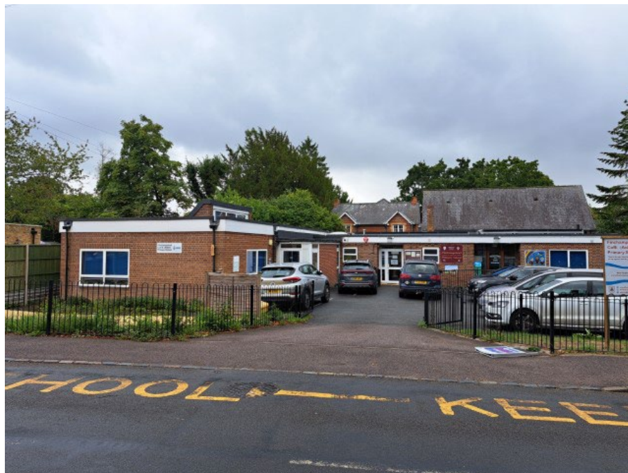
Photo 1 – View of front elevation (north)
