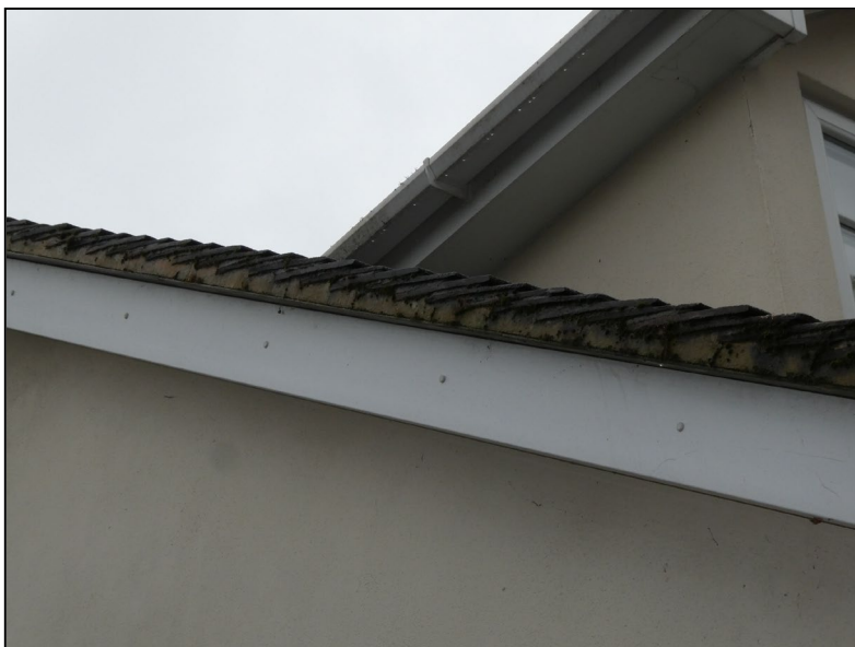
Figure 7. Example sealed uPVC soffits and fascias. 412 Finchampstead Road, Wokingham. 14.11.25
