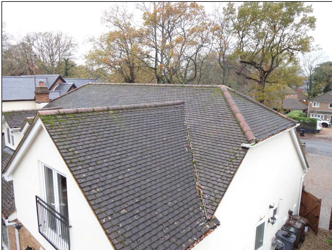
Figure 4. Example well fitted roof tiles. 412 Finchampstead Road, Wokingham. 14.11.25
