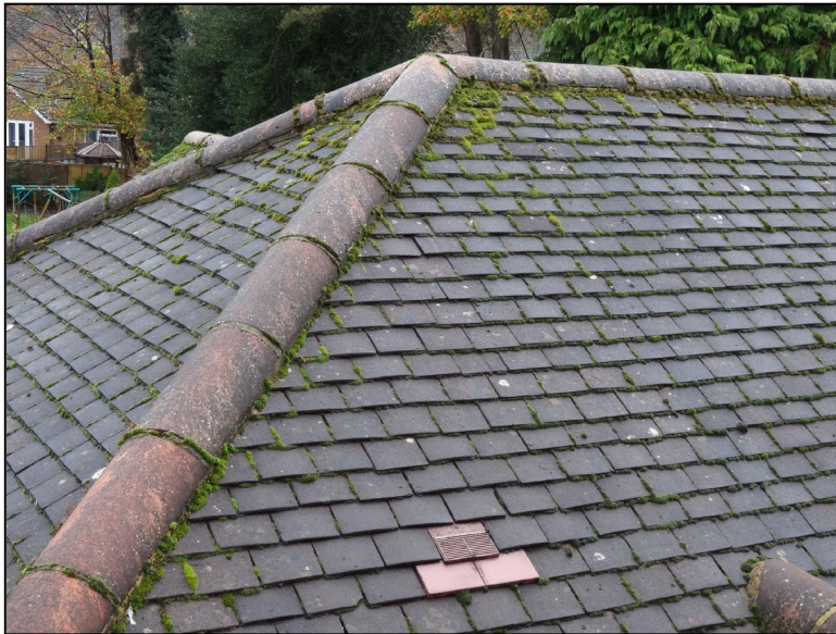
Figure 6. Example sealed verge. 412 Finchampstead Road, Wokingham. 14.11.25
