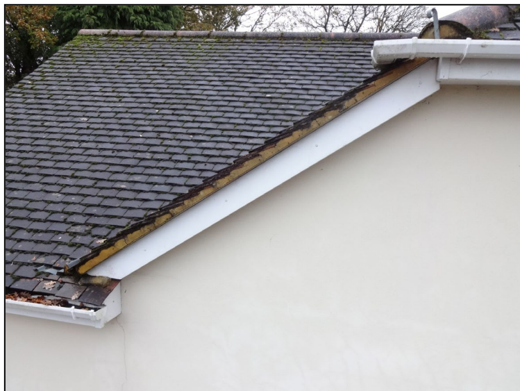
Figure 7. Example sealed uPVC soffits and fascias. 412 Finchampstead Road, Wokingham. 14.11.25
