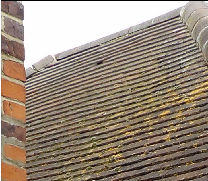
Figure 5. Missing roof tile and missing mortar. Blackmoor, Three Mile Cross. 02.09.25
