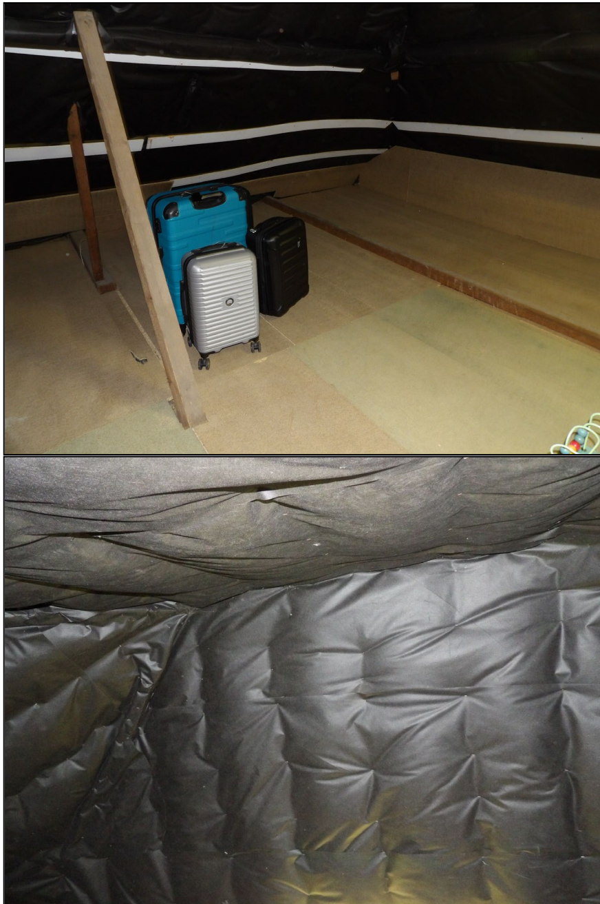
Figure 11. Example of loft space and unlined roof tiles. Blackmoor, Three Mile Cross. 02.09.25
