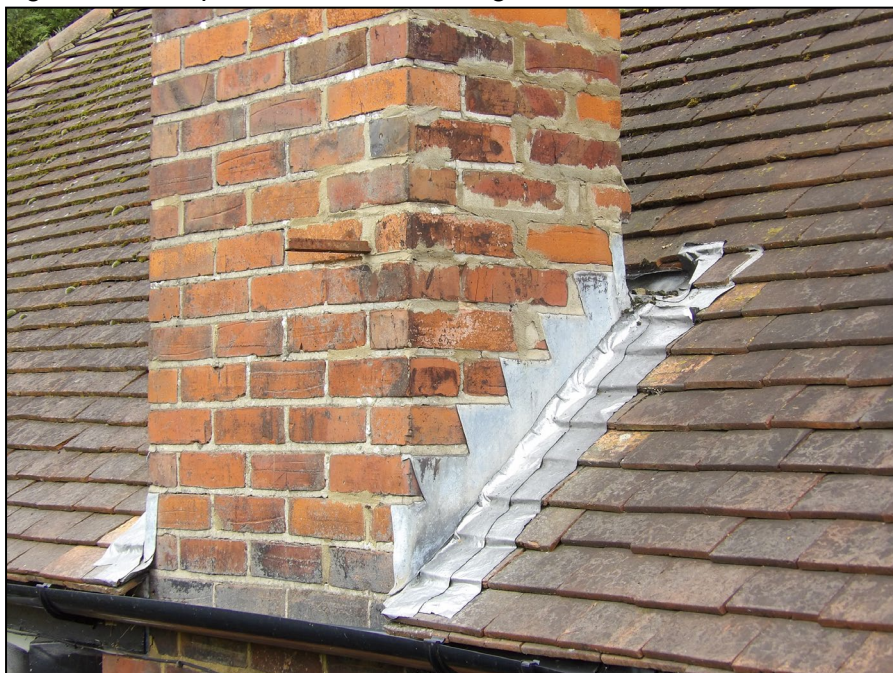
Figure 8. Example sealed lead flashing. Blackmoor, Three Mile Cross. 02.09.25
