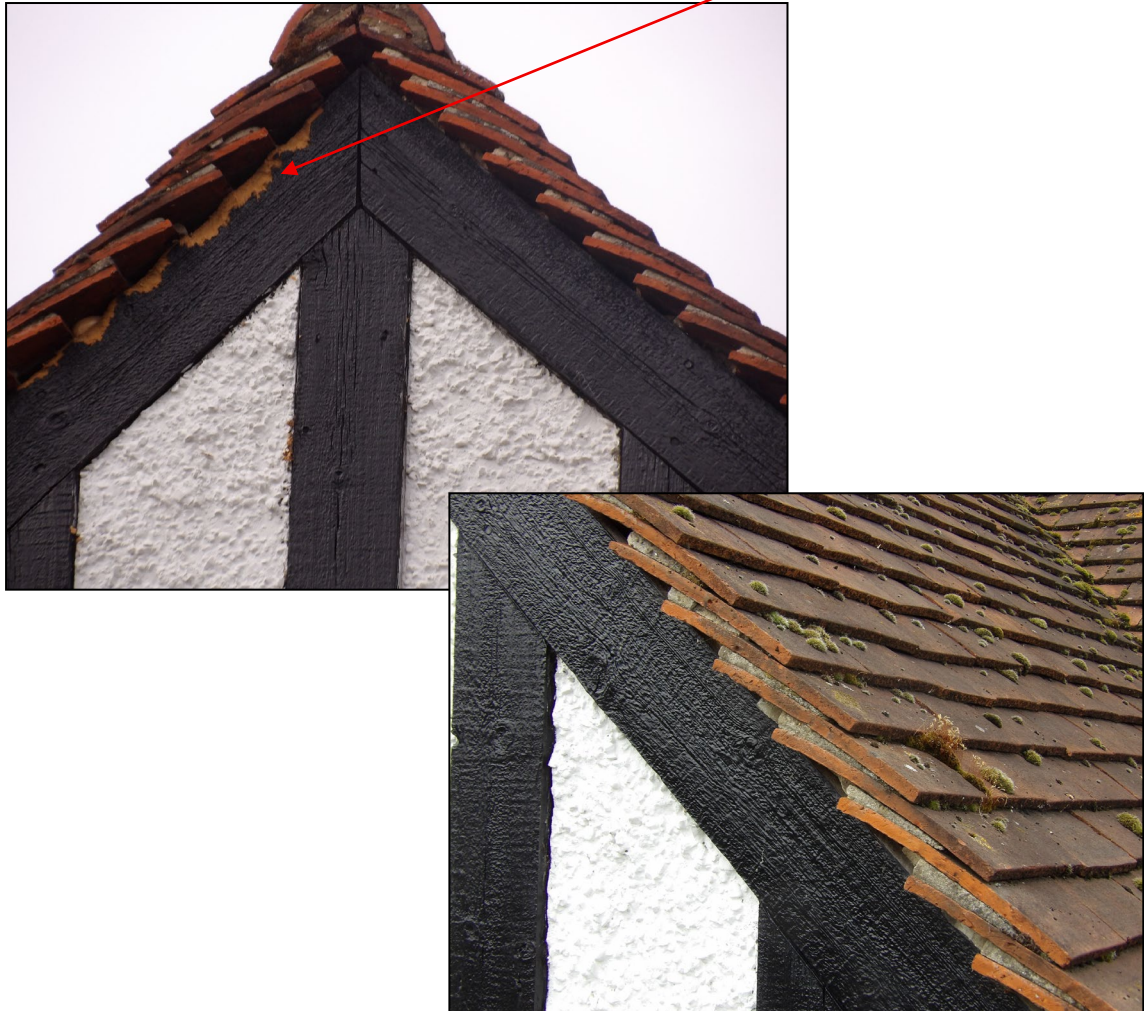
Figure 8. Example sealed lead flashing. Blackmoor, Three Mile Cross. 02.09.25
