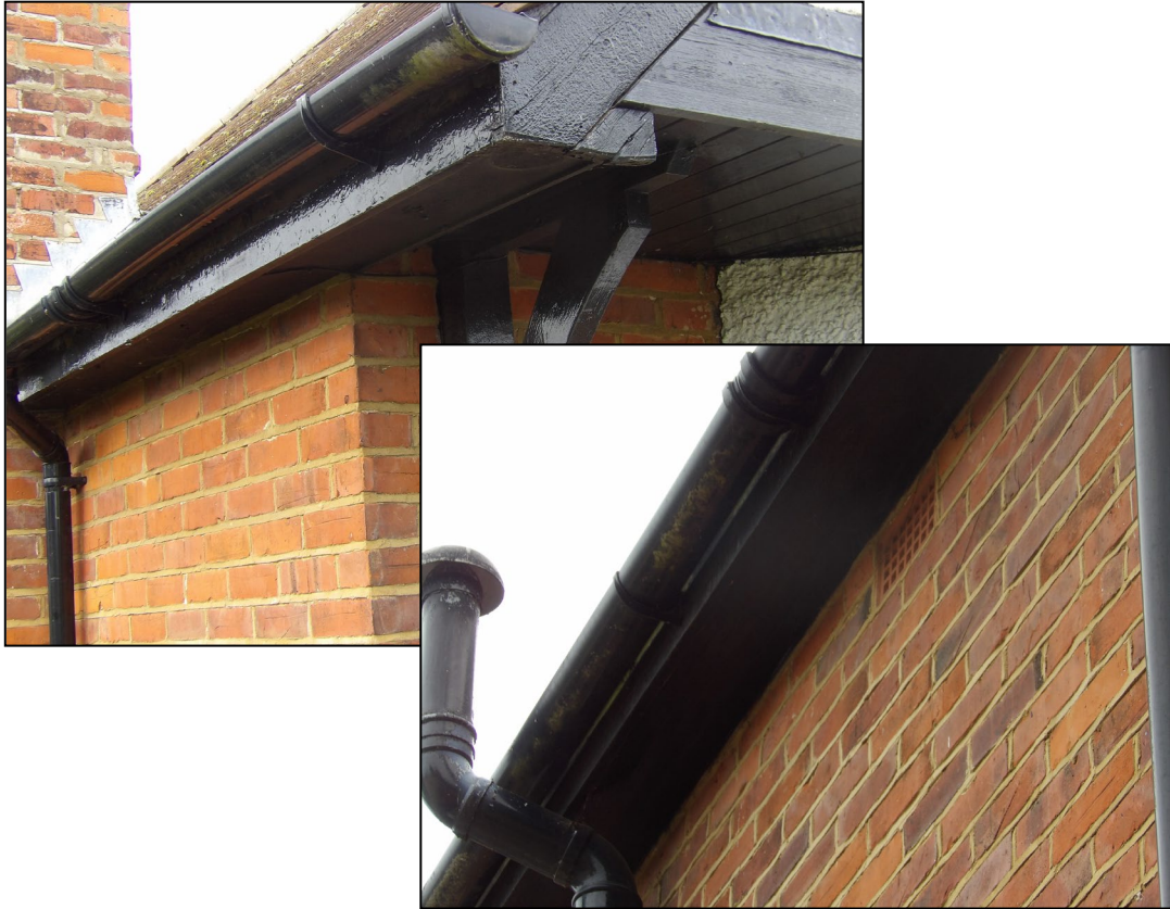
Figure 9. Example sealed soffits/fascias. Blackmoor, Three Mile Cross. 02.09.25
