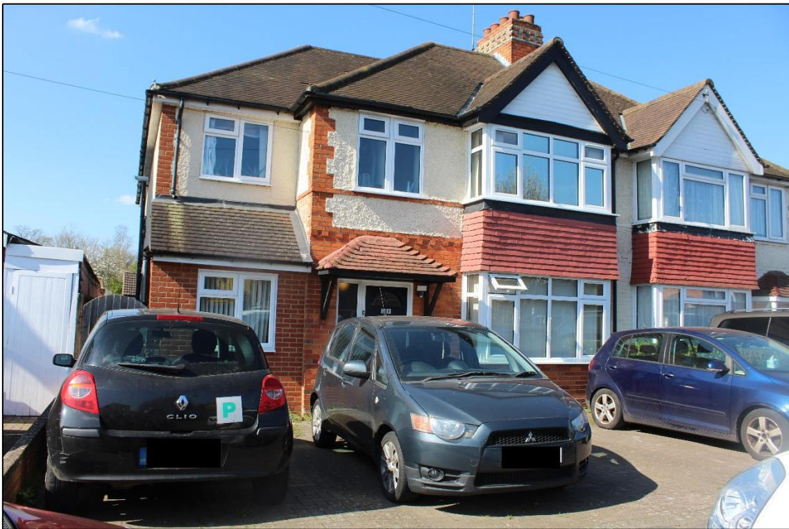
Photograph 1 – Front elevation as viewed from the pavement
