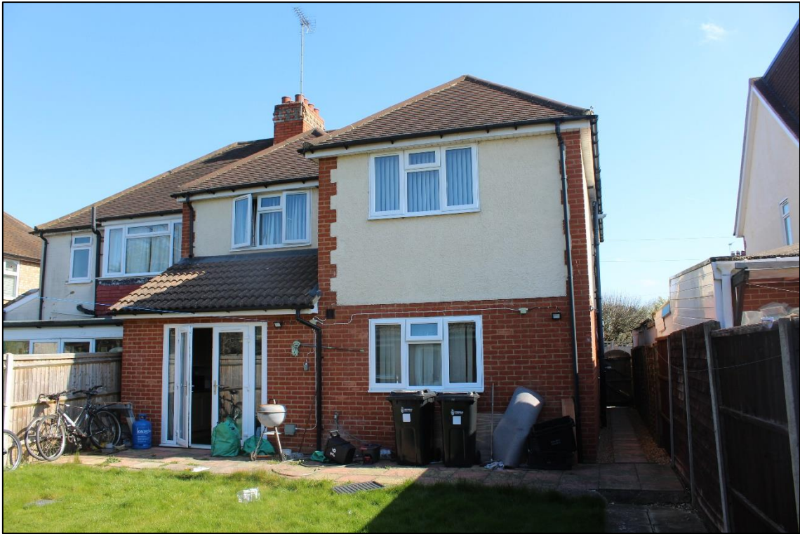
Photograph 2- Rear elevation as viewed from the garden
