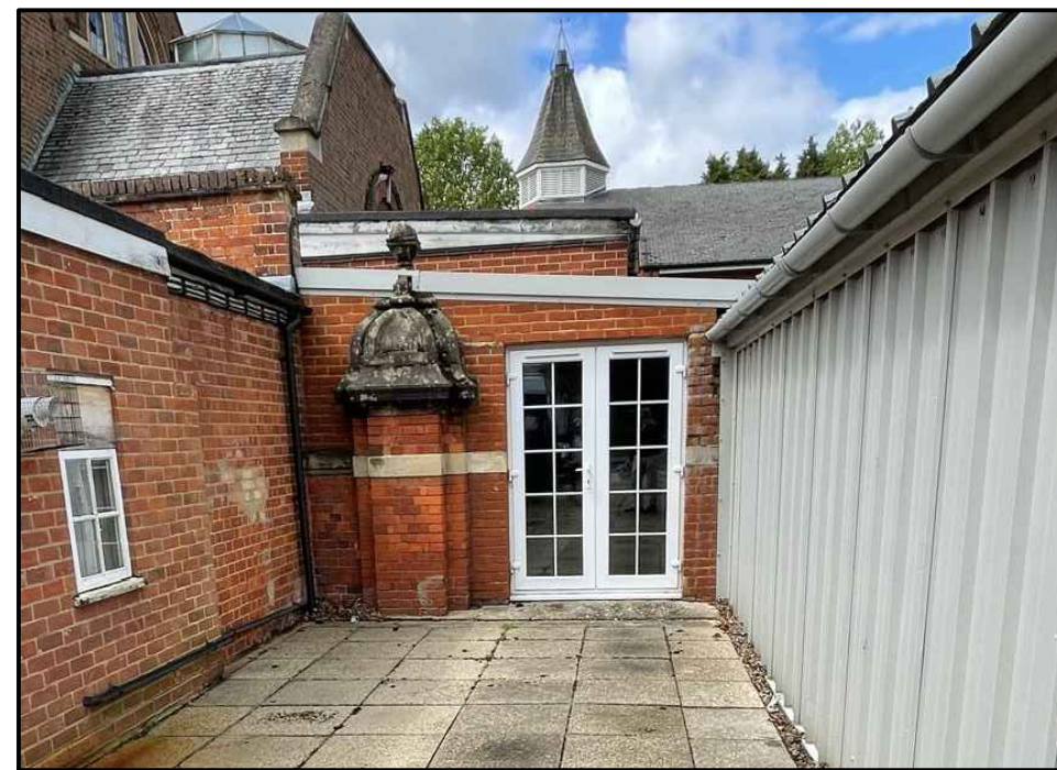
EXTERNAL VIEW OF BRICK PIER
