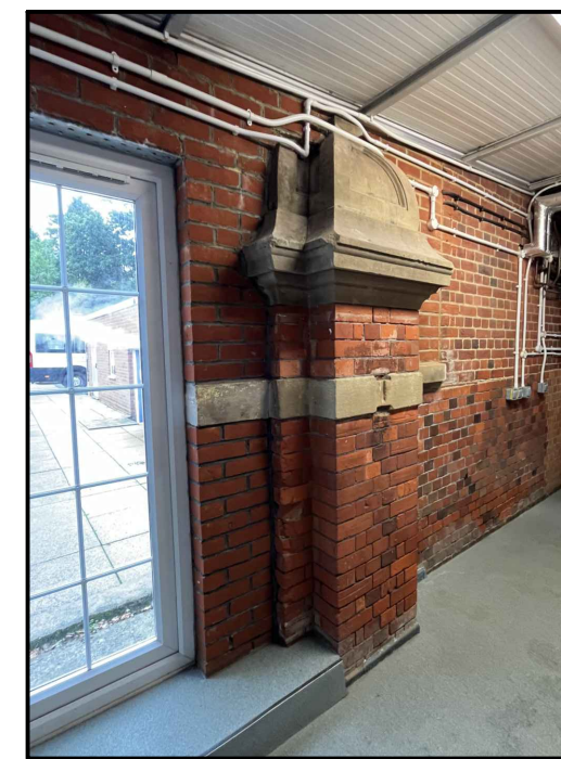
INTERNAL VIEW OF BRICK PIER
