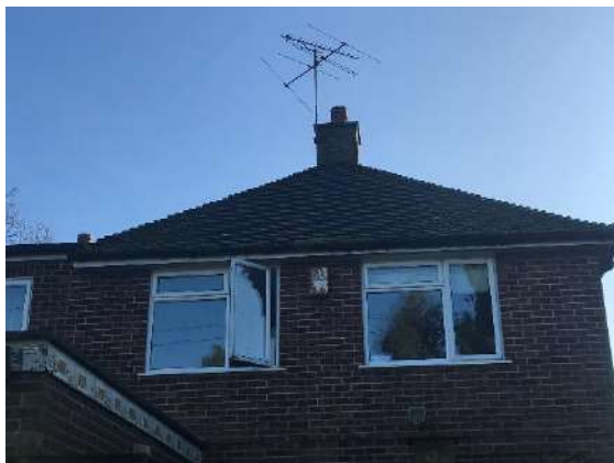
Photograph 3: Overview of No.87 roof structure.
