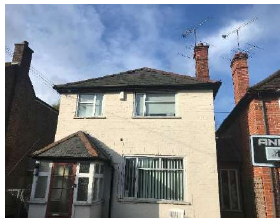
Photograph 6: Overview of No.85.
