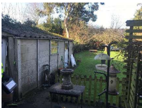
Photograph 5: Back garden of No.87.
