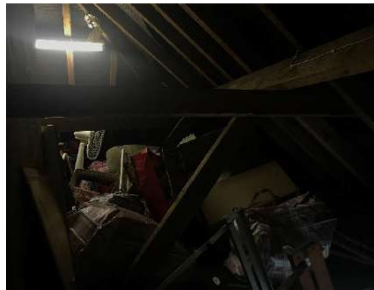
Photograph 4: No. 87 cluttered roof void.
