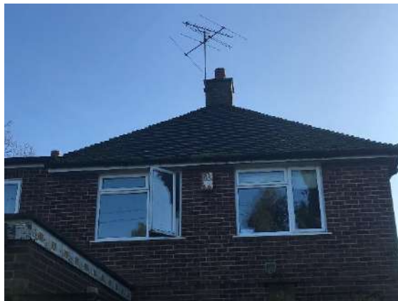
Photograph 3: Overview of No.87 roof structure.
