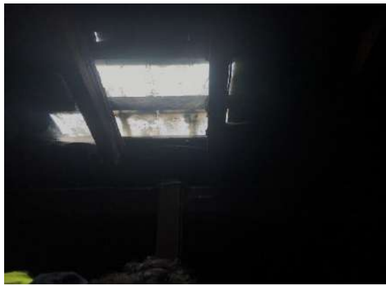
Photograph 7: Skylight in No.85 roof void, lots of daylight ingress.
