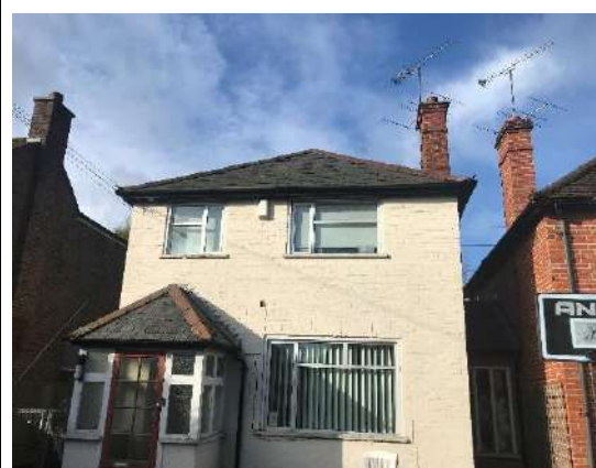
Photograph 6: Overview of No.85.
