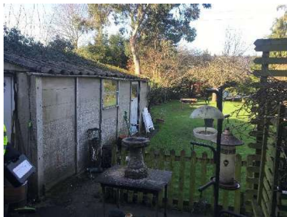
Photograph 5: Back garden of No.87.
