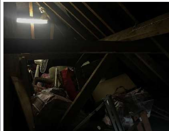
Photograph 4: No. 87 cluttered roof void.
