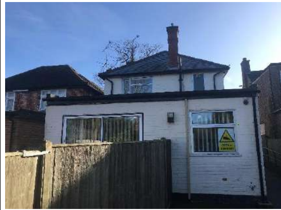
Photograph 8: Rear view of No.85.
