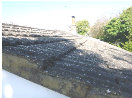
Photograph 4. Interlocking roof, ridge and hip tiles intact.
