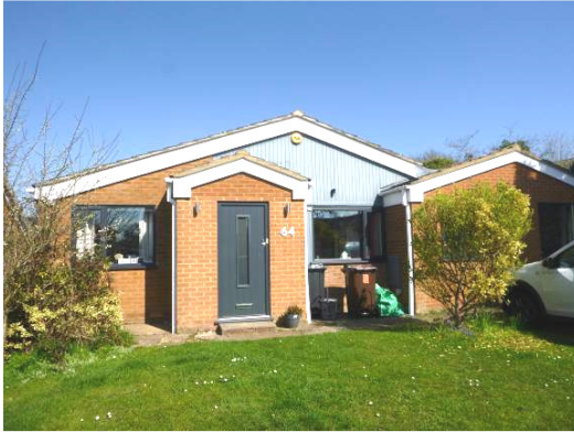
Photograph 1. Front of property viewed from south.
