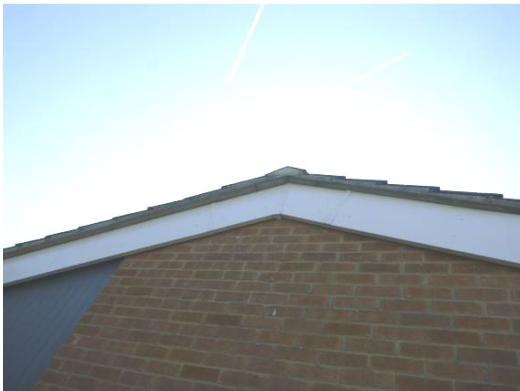
Photograph 5. Verge mortar intact throughout.
