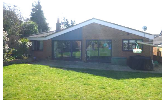
Photograph 2. Rear of property viewed from north.
