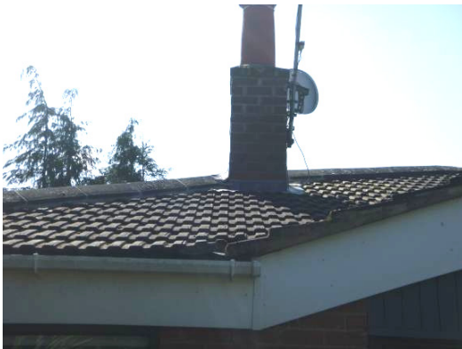
Photograph 3. Interlocking roof, ridge and hip tiles intact.
