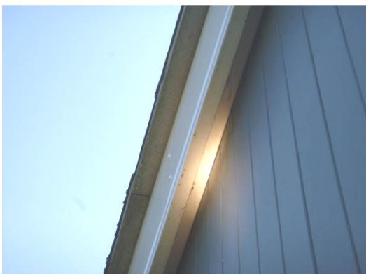
Photograph 9. Fascias tight to walls on other elevations, cladding flat and tight.
