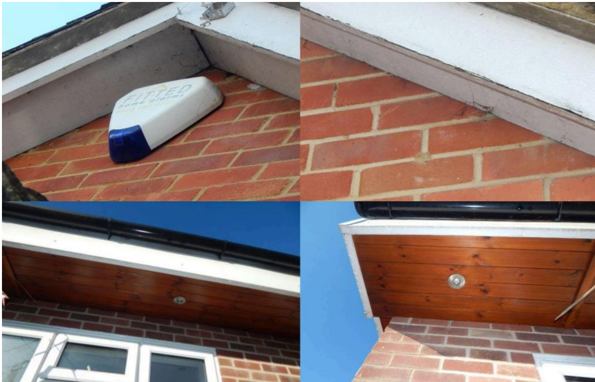
Image 4 – Close view of eaves coverings which have demonstrated a fair condition throughout
