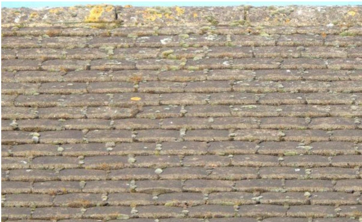
Image 5 – Close view of tiled roof coverings to demonstrate condition throughout
