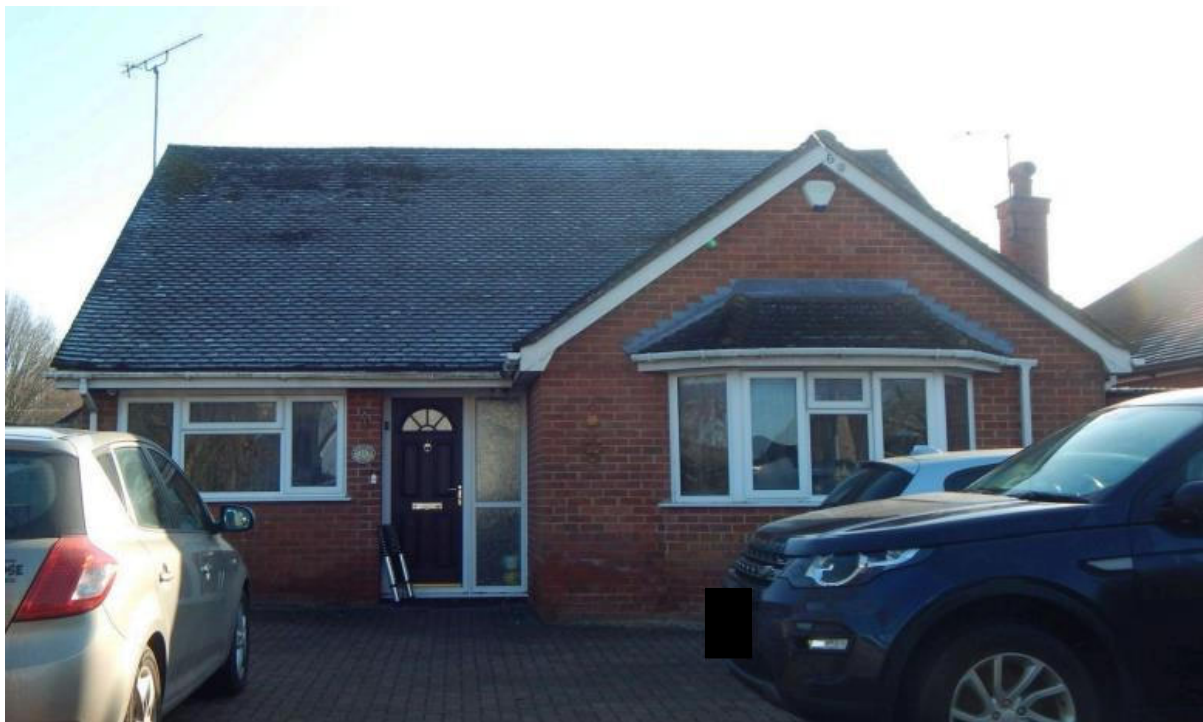
Image 1 – West facing elevation of the property
