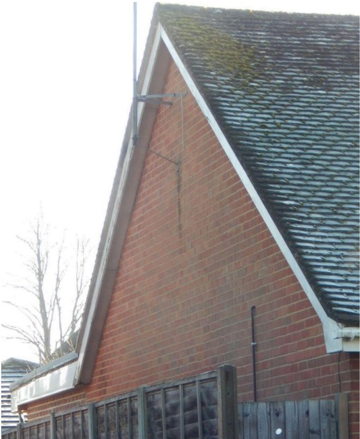
Image 3 – North facing elevation of the property
