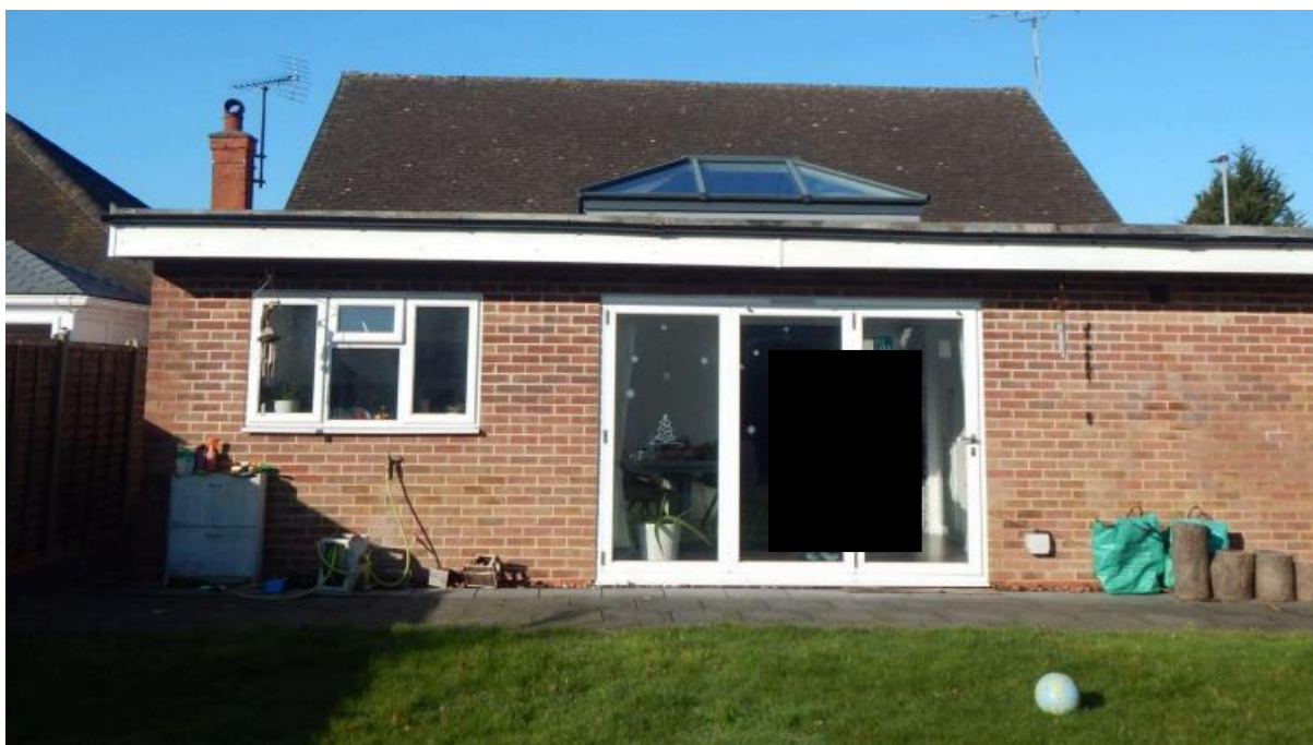
Image 2 – East facing elevation of the property
